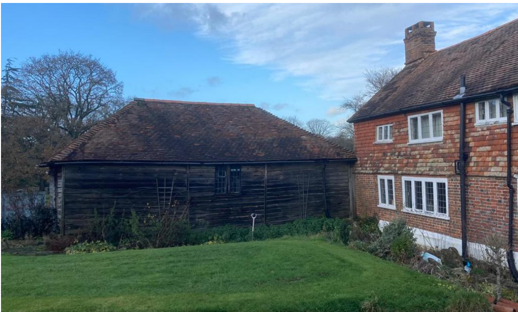
The Granary rear (SE) elevation.
