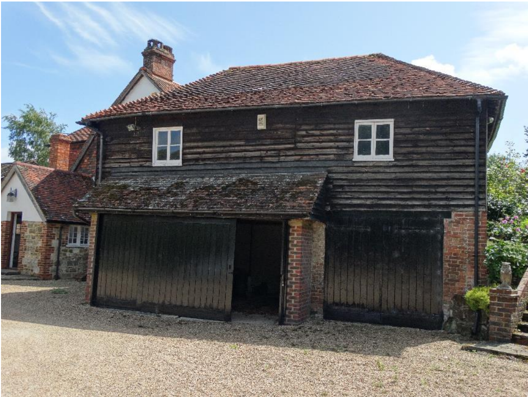
The Granary front (NW) elevation.
