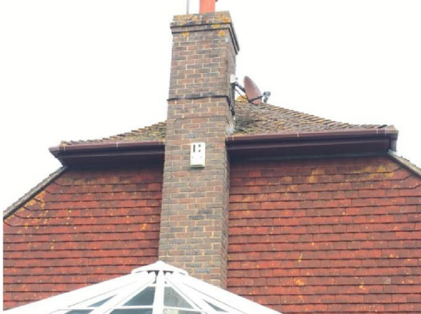
Many hanging tiles in good condition
