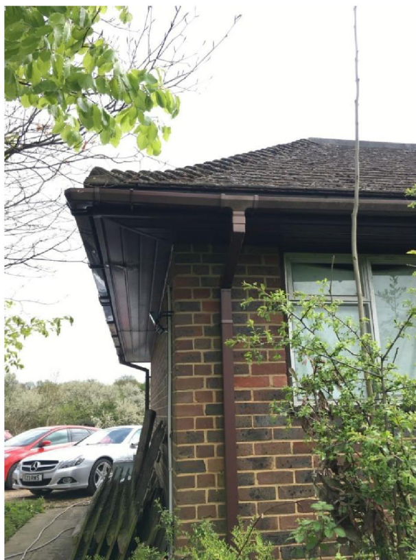
Garage in good condition, no access points for bats
