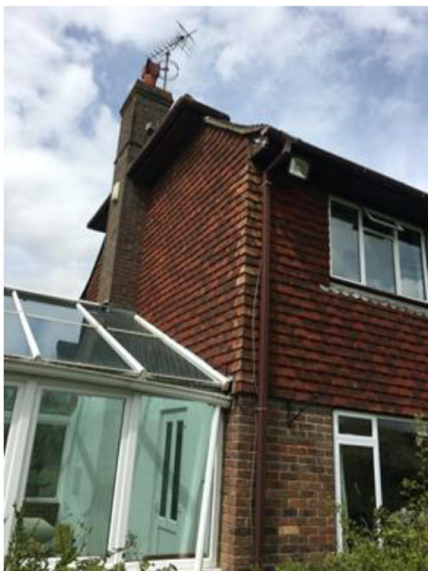
Brickwork in good condition
