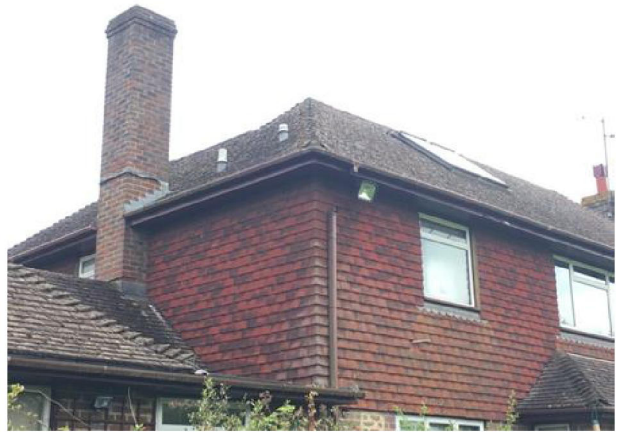
Tightly fitting lead flashing to the window, drainage pipe
