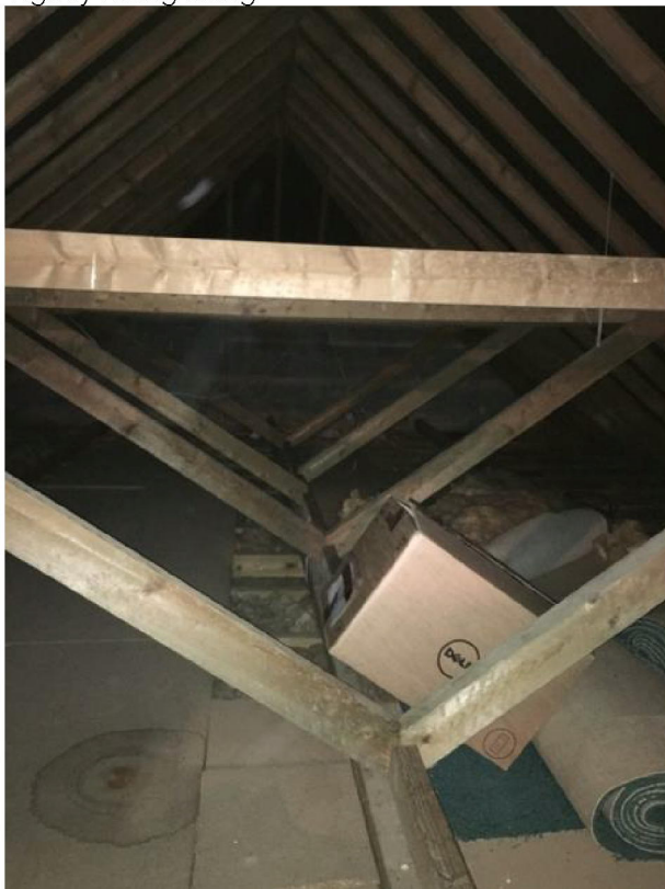
Internal flight space, some cross beams
