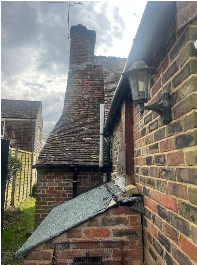
Rear roof pitch
