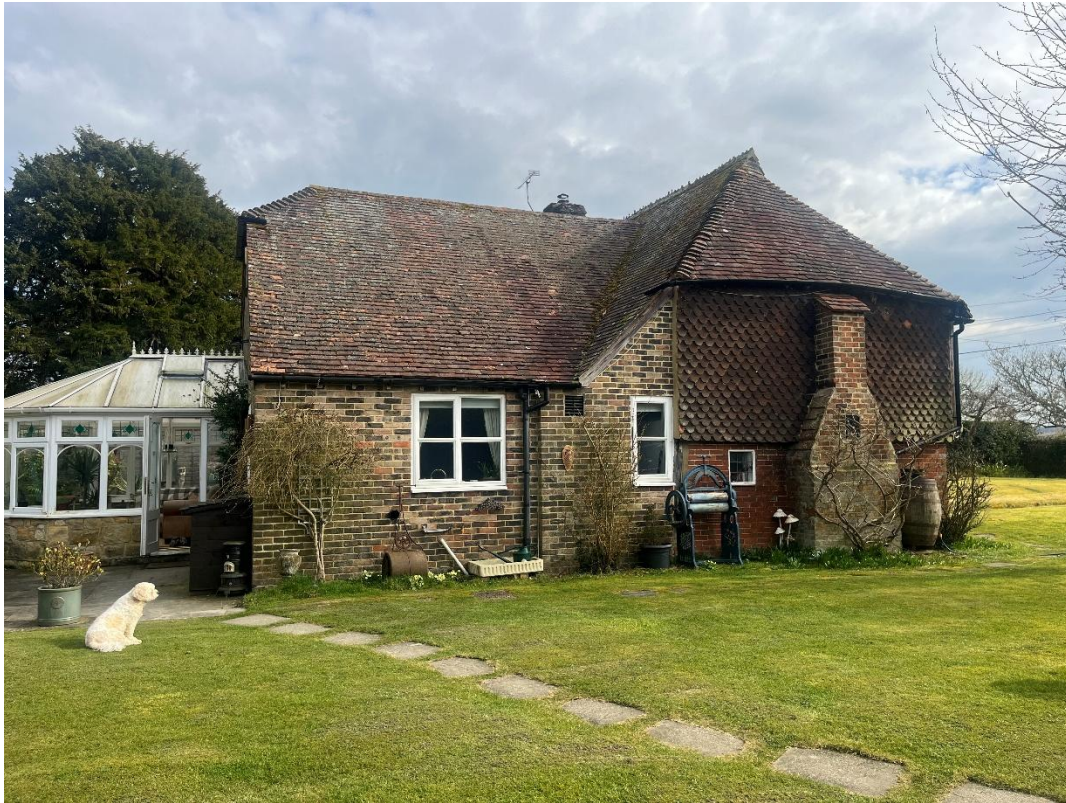
Side of property showing side and rear roof pitches
