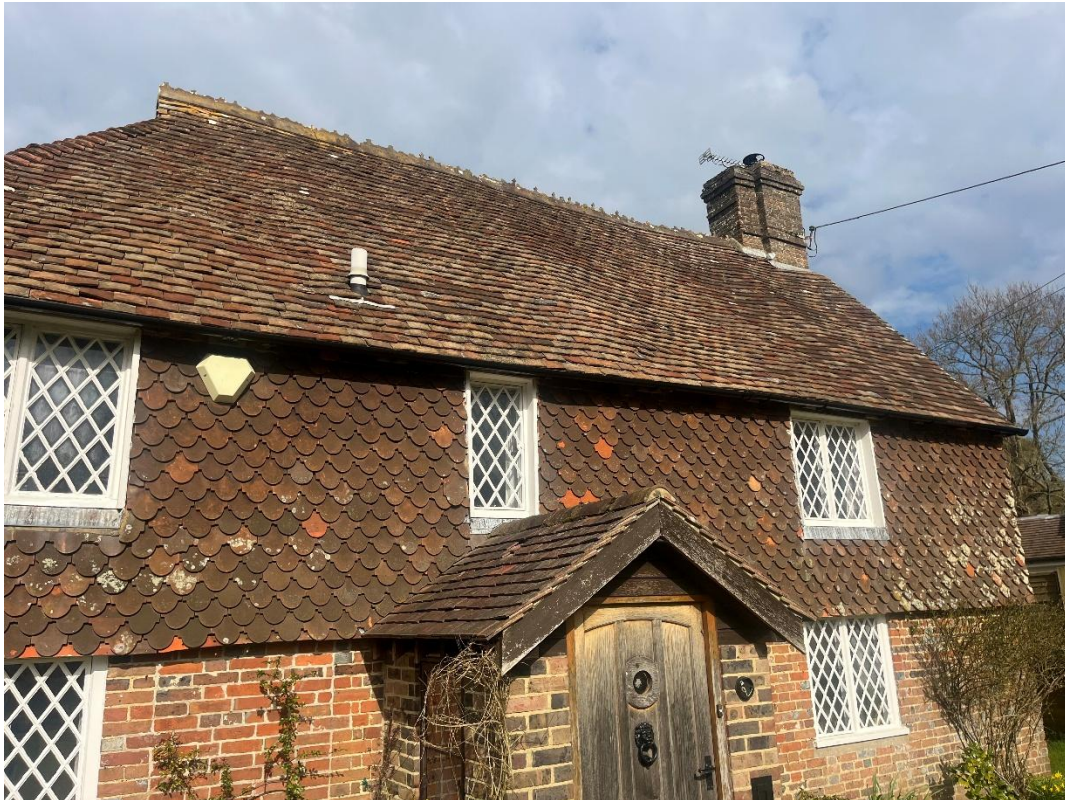
Front of property showing front roof pitch and porch roof.
