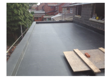
Flat roof - EPDM Rubber
