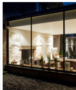
Glazing Windows, Doors, Lantern Rooflight, and roof coping- PPC aluminium slimline double glazed units, RAL 7016, Anthracite Grey
