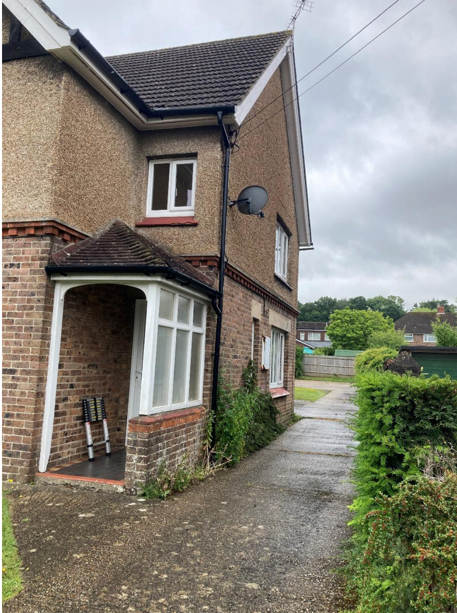
Image 02 – External side access between no. 12 and the South-Eastern boundary
