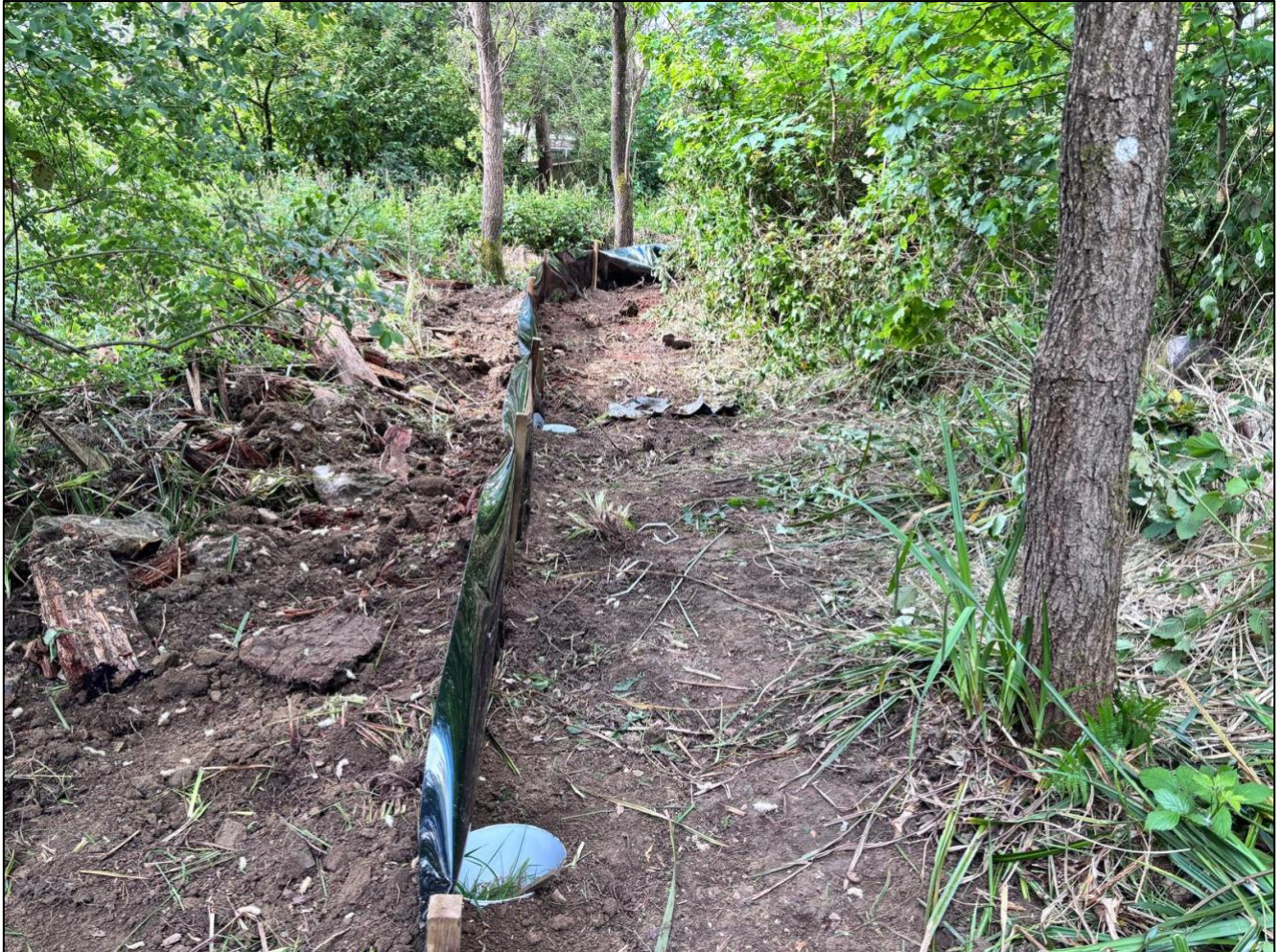
Photograph 2. A photo taken on 12.05.26 showing the temporary amphibian fencing installed at Land at Parklands.
