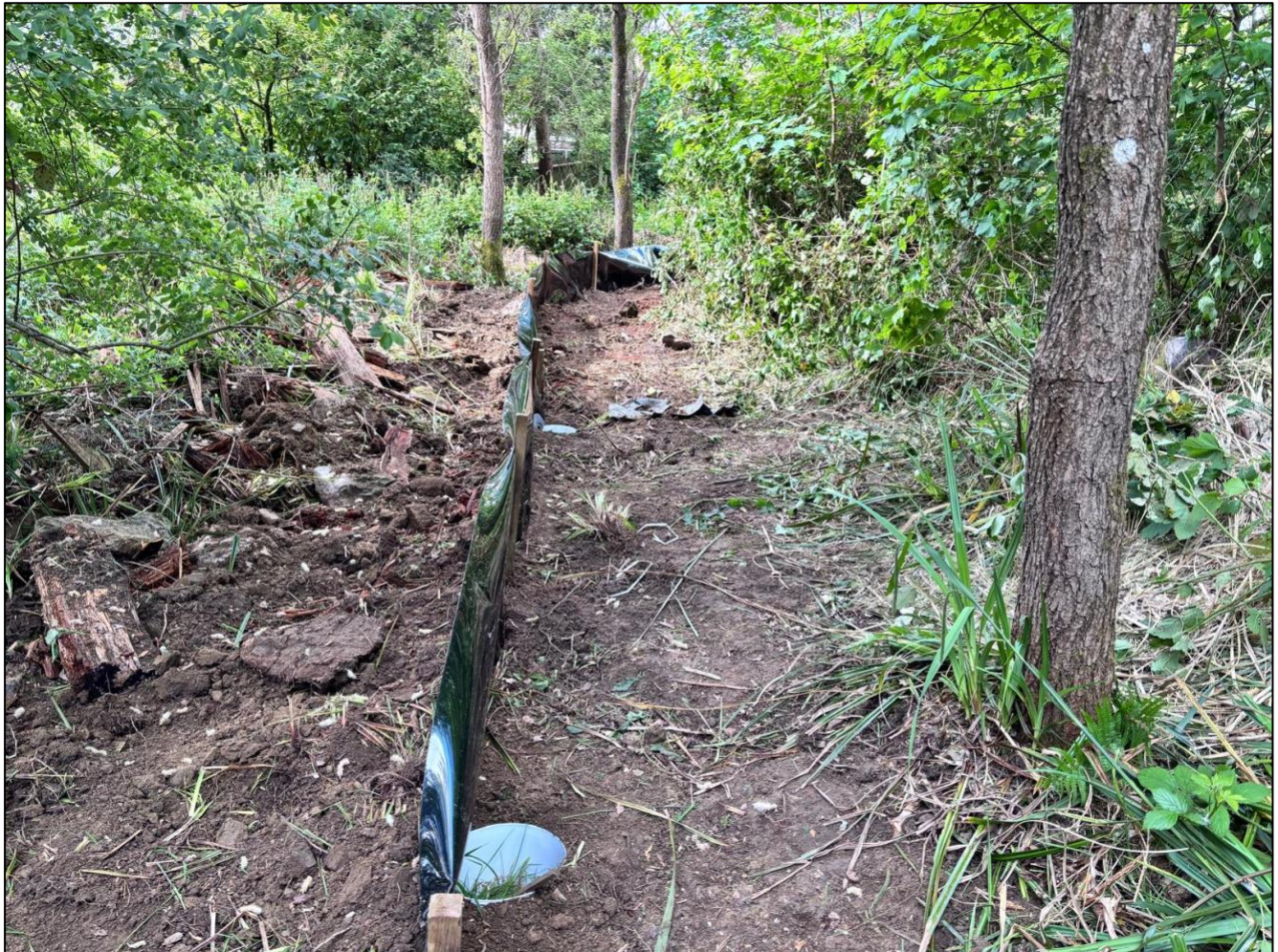
Photograph 1. A photo taken on 12.05.26 showing the temporary amphibian fencing installed at Land at Parklands.
