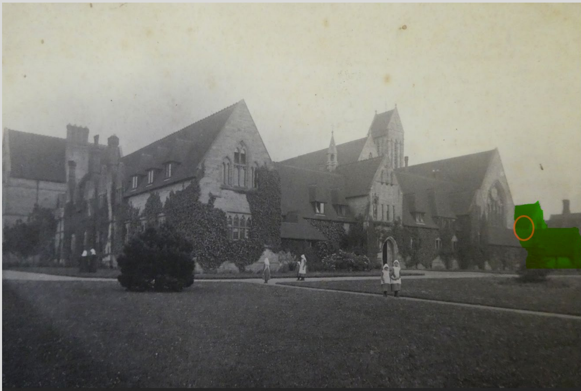
Image 1 – Photo of Convent showing No 17 in green. A straight parapet profile can be seen within the orange circle
