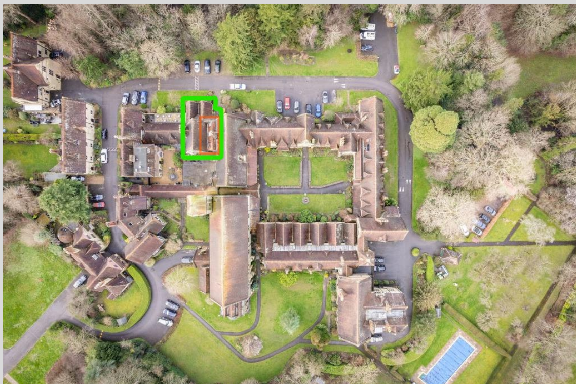
Image 4 - Current aerial/drone view showing the visibly different tile covering to the later secondary roof within the wider roofscape. No 17 is bounded in green with the secondary roof bounded orange.
