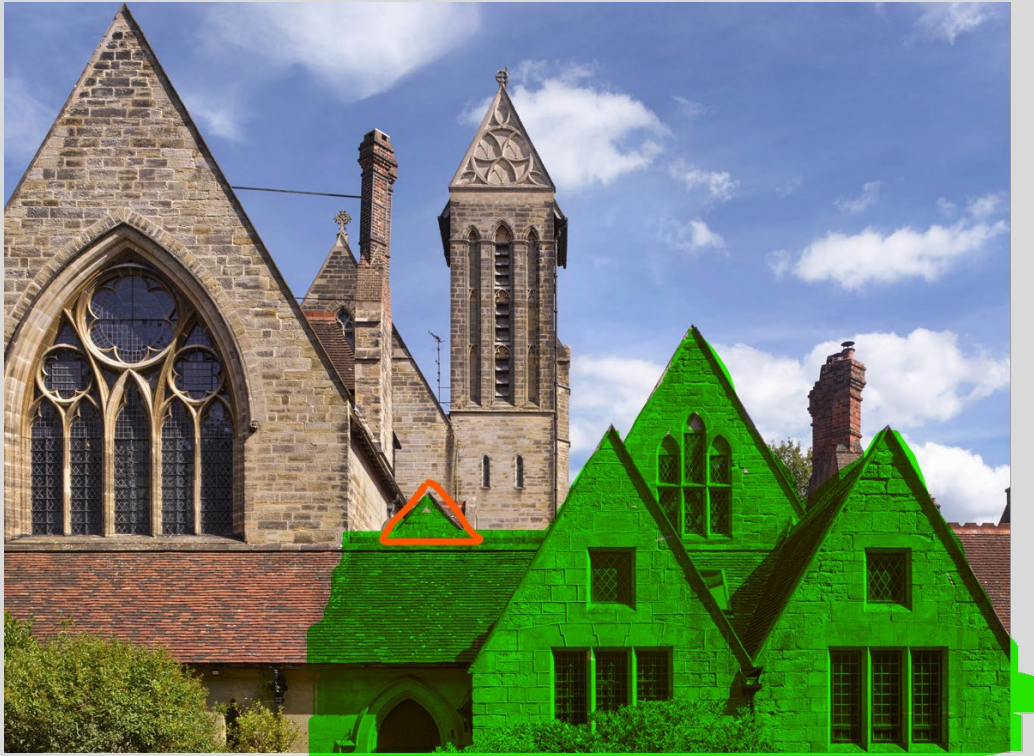
Image 2 - Current photo of the front of No 17 shown in green. The 1970's introduction of the raised secondary roof is highlighted orange
