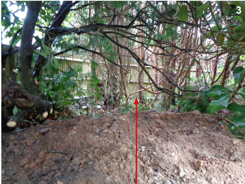
G7 Cypress to be removed.
