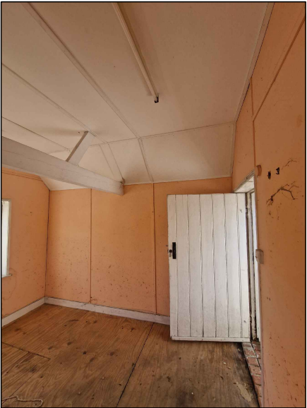
Interior photo of existing ceiling in 1950s extension block
