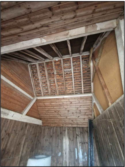
Interior photo of existing bay in former stable
