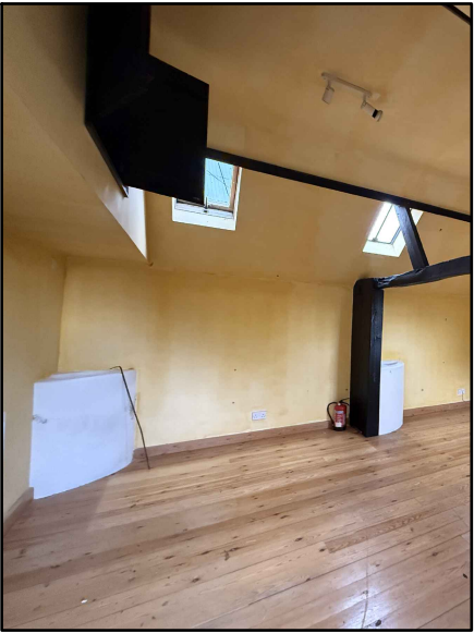
Interior photo of existing timber floor (portion) & plasterboard wall finish (portion) in existing recreation area within former stable
