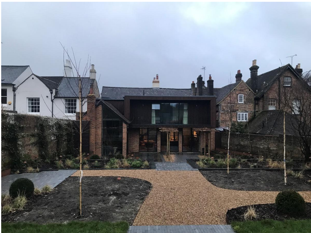
Figure 32: View of Marlow House from the rear garden (west). Note the prominence of the restored 15 th century roofscape compared to the prior situation shown at Figure 7.
