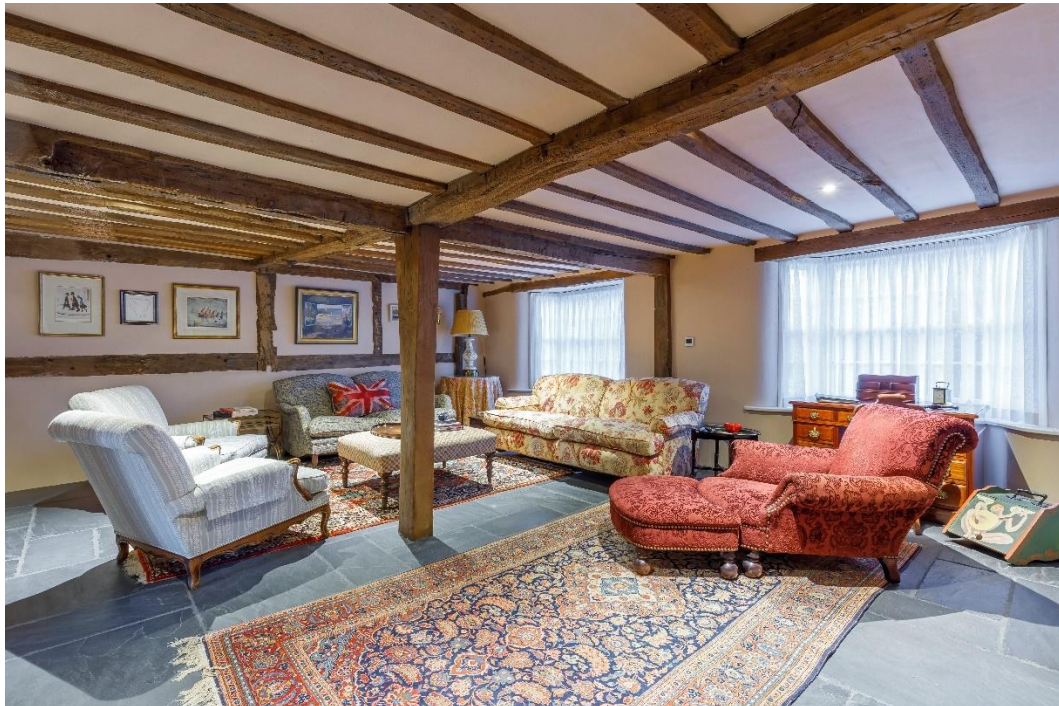
Figure 15: Supporting timber post in seasoned oak as implemented
