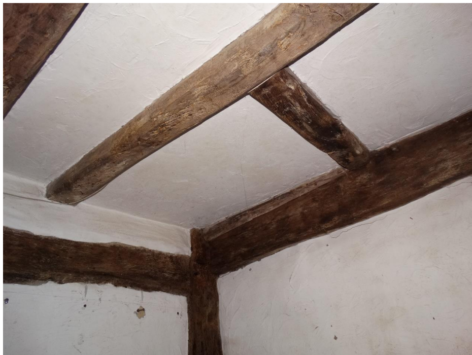
Figure 10: Corner trimming for a ladder stair hole in the northwest corner and this is considered to be original. Source: Desbruslais Chartered Surveyors Statement of Heritage Significance of 13 th October 2022
