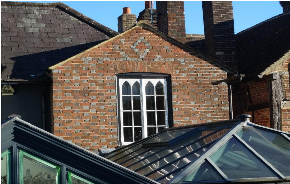
Figure 17: 1830s gabled outrigger with vitrified blue brick header detailing. Source: Desbruslais Chartered Surveyors Statement of Heritage Significance of 13 th October 2022
