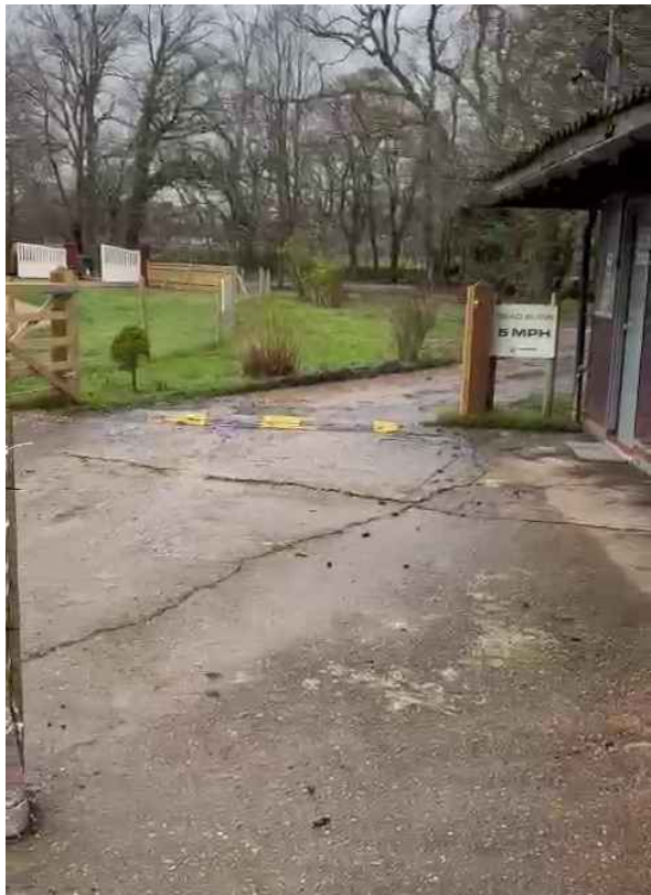
1. Facing west towards existing Wintons Fishery access
