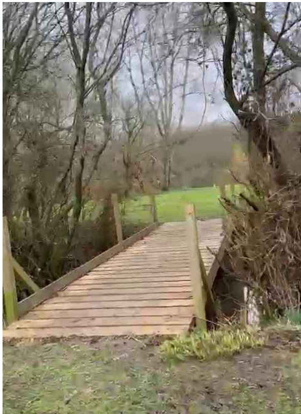
10. West across existing footbridge between Heron Lake and Kingfisher Lake
