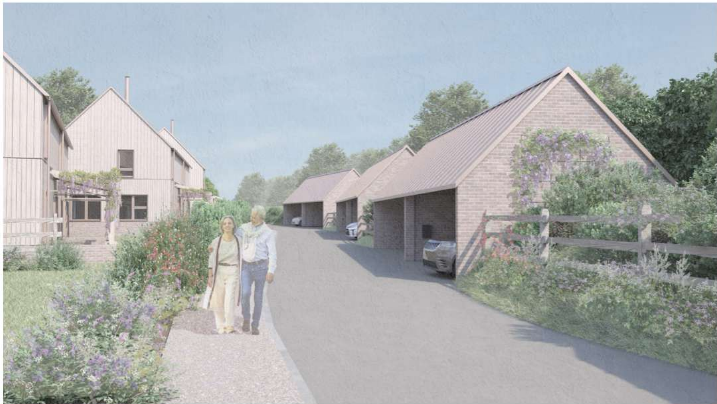
View 01. Looking North up the access road.
