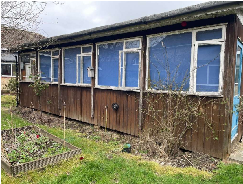
Figure 2 : The building to be demolished
