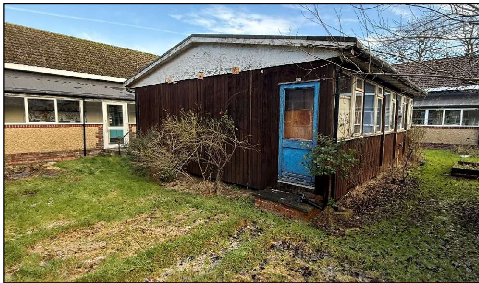
Figure 3 Existing dilapidated classroom to be demolished (Looking West).
