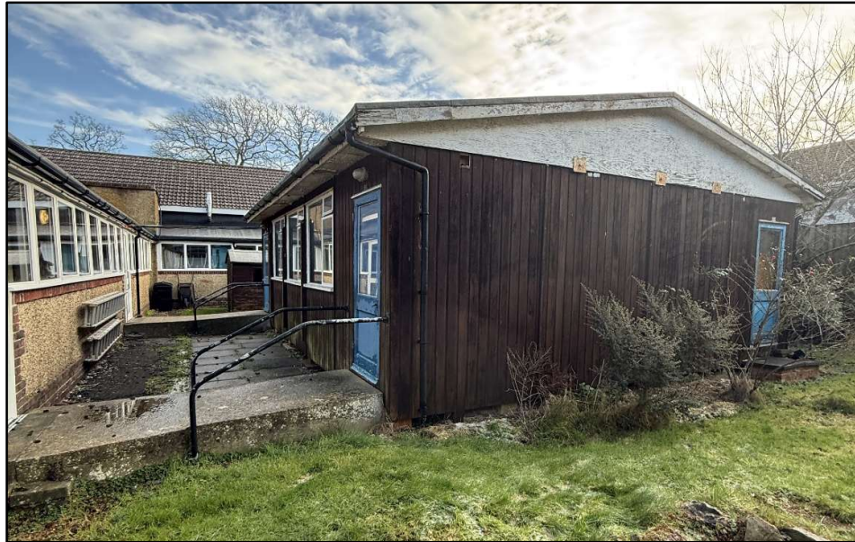
Figure 4 Existing classroom to be demolished (Looking East).
