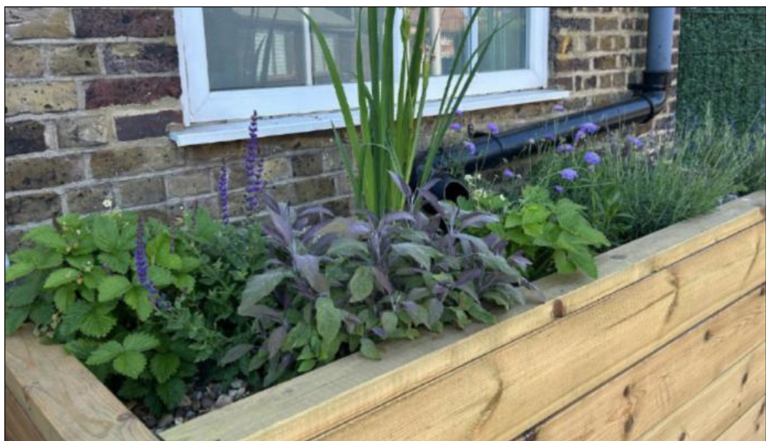
Figure 4.2 SuDS Planter installation (Meristem Design 2026)
