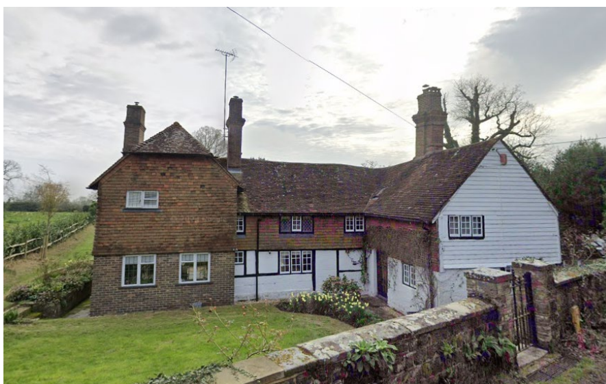
Figure 3.9: Durstons (Source – Google Streetview).
