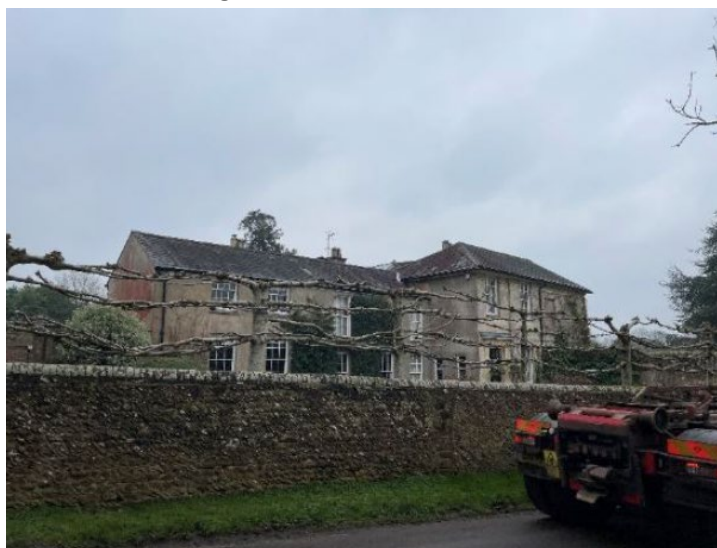
Figure 3.22: Bolney Lodge from Foxhole Lane (Source – Pegasus Heritage Statement).
