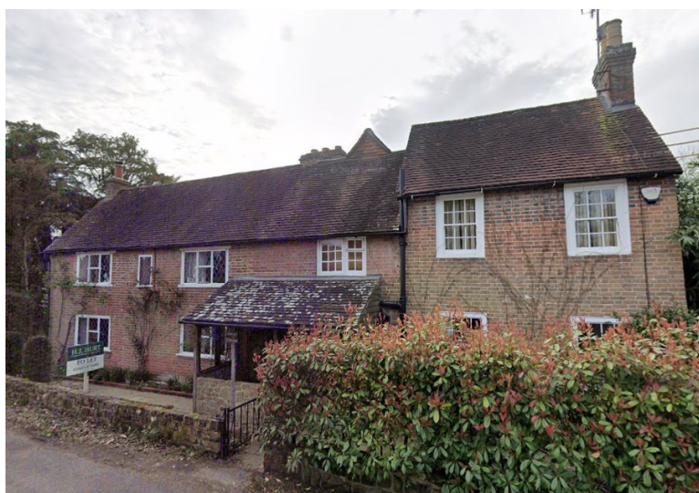
Figure 3.26: Bolney Lodge Cottage – the taller element to the right side is the later cottage (Source – Google Maps).
