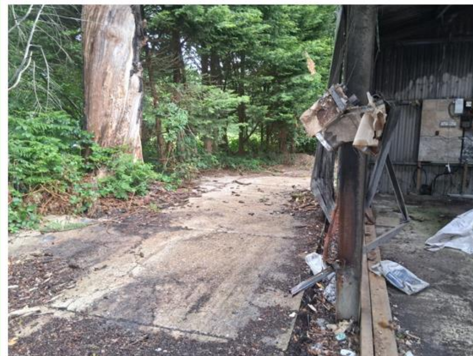
Photo No.6: Facing SE showing the NE face of barn and the hardstanding area adj. to this face of the barn
