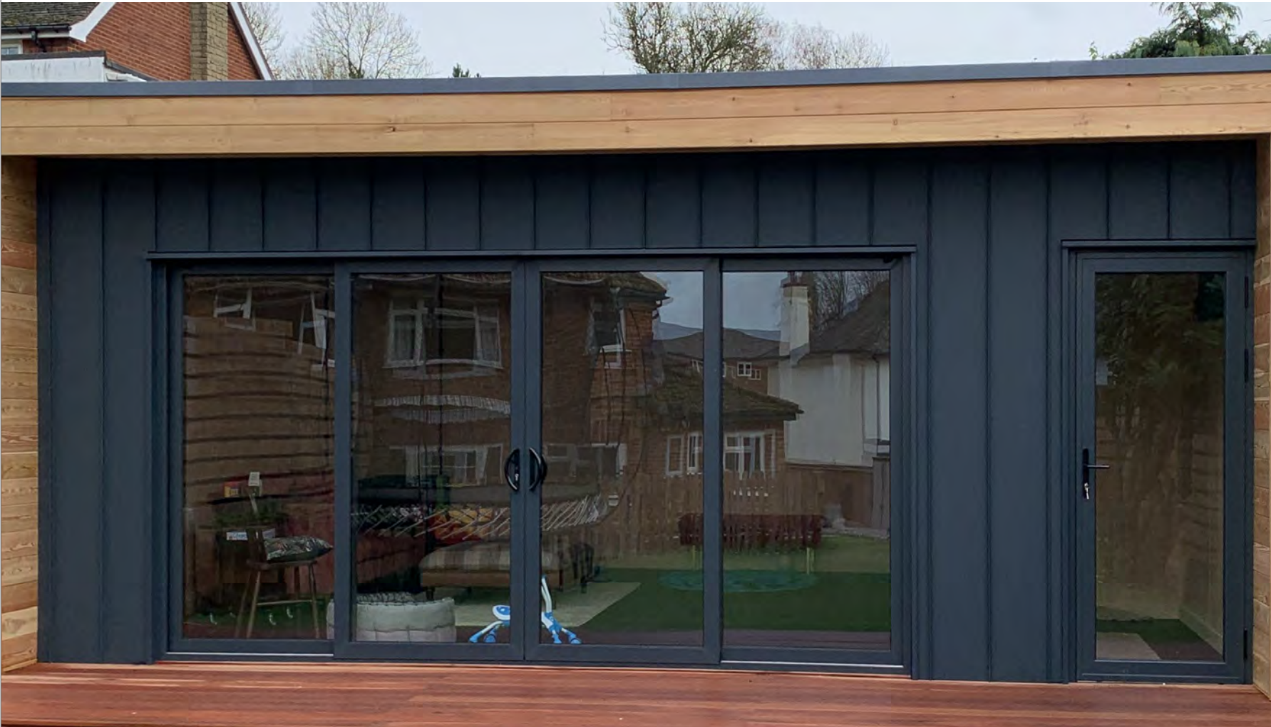
25mm Standing Seam Sheet Metal Rainscreen
