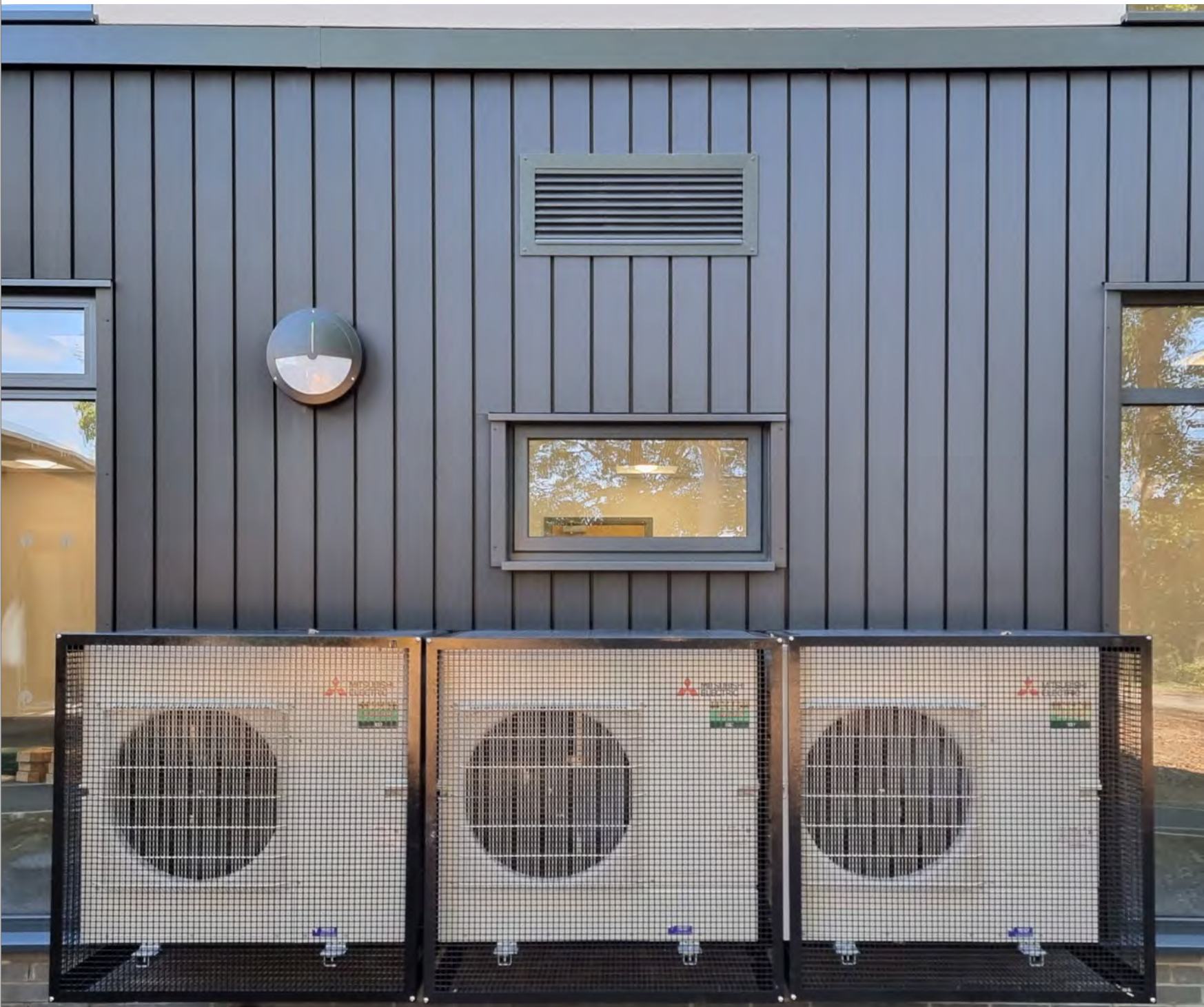
Mitsubishi Air Source condenser unit (factory finish) with protective guard, powder coated to RAL7016 to match windows and door finish (note placement is indicative and subject to alteration by specialist)
