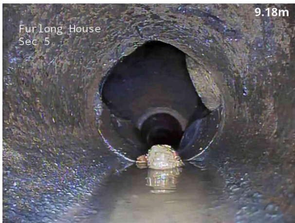
11, 00:01:59, 9.35 m Finish node, manhole, reference: EXFMH1403b
