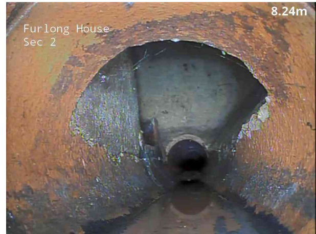
2, 00:01:36, 8.34 m Finish node, manhole, reference: F08a
