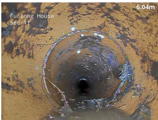
3, 00:00:47, 6.15 m Roots, fine at joint
