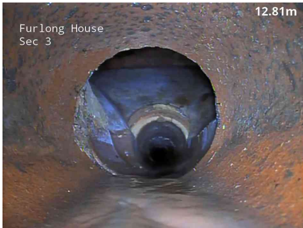
3, 00:01:43, 13.00 m Finish node, manhole, reference: EXFMH1403
