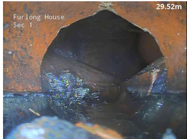
8, 00:05:34, 30.00 m Finish node, manhole, reference: EXFMH1403b
