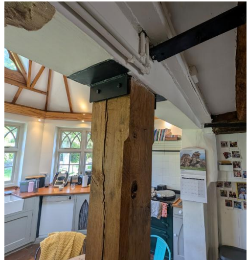
Figure 6 - Existing timber post
