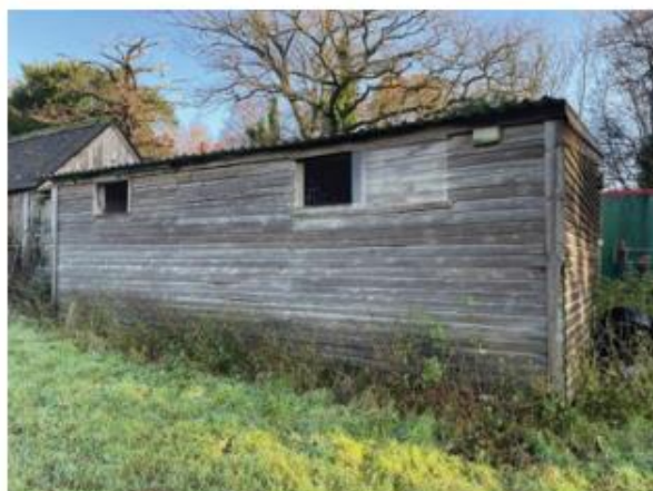
Western elevation of B6.
