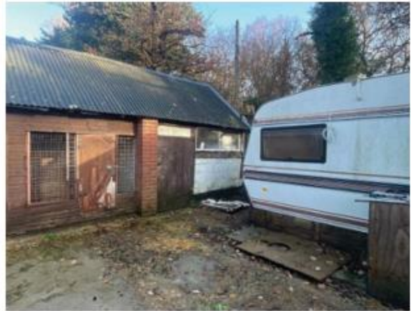
South eastern elevation of B2.
