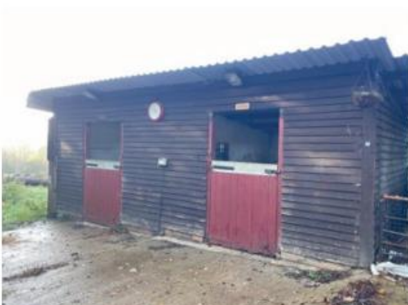
Eastern elevation of B6.
