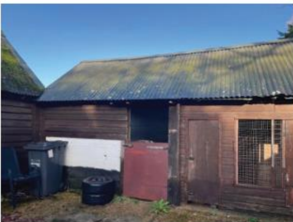
Open access into western section of B2.
