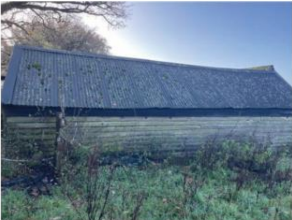
Northern elevation of B2.
