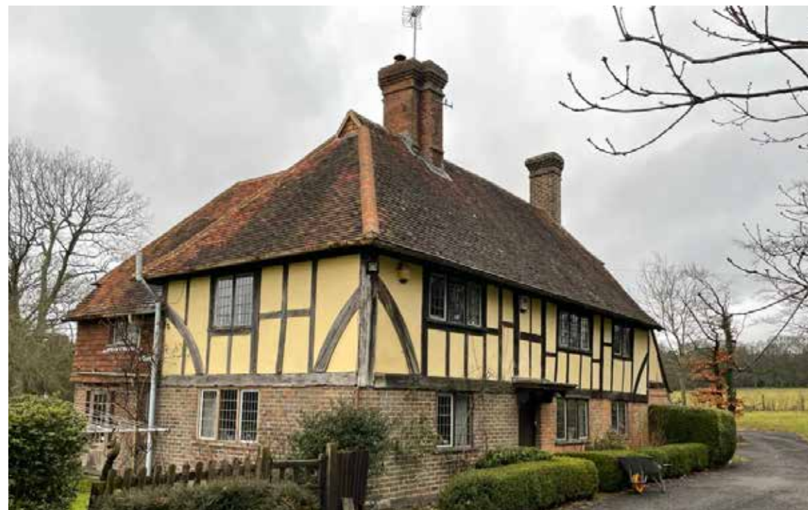
Grade II listed Kings Farmhouse, some 850m from the site
