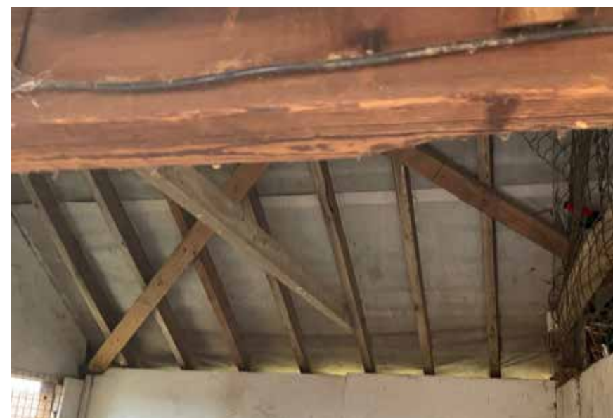
Existing internal rafters
