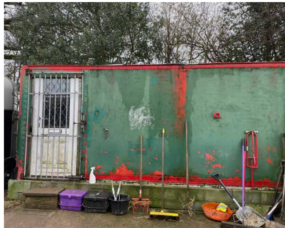
Existing storage structure and caravan to be removed
