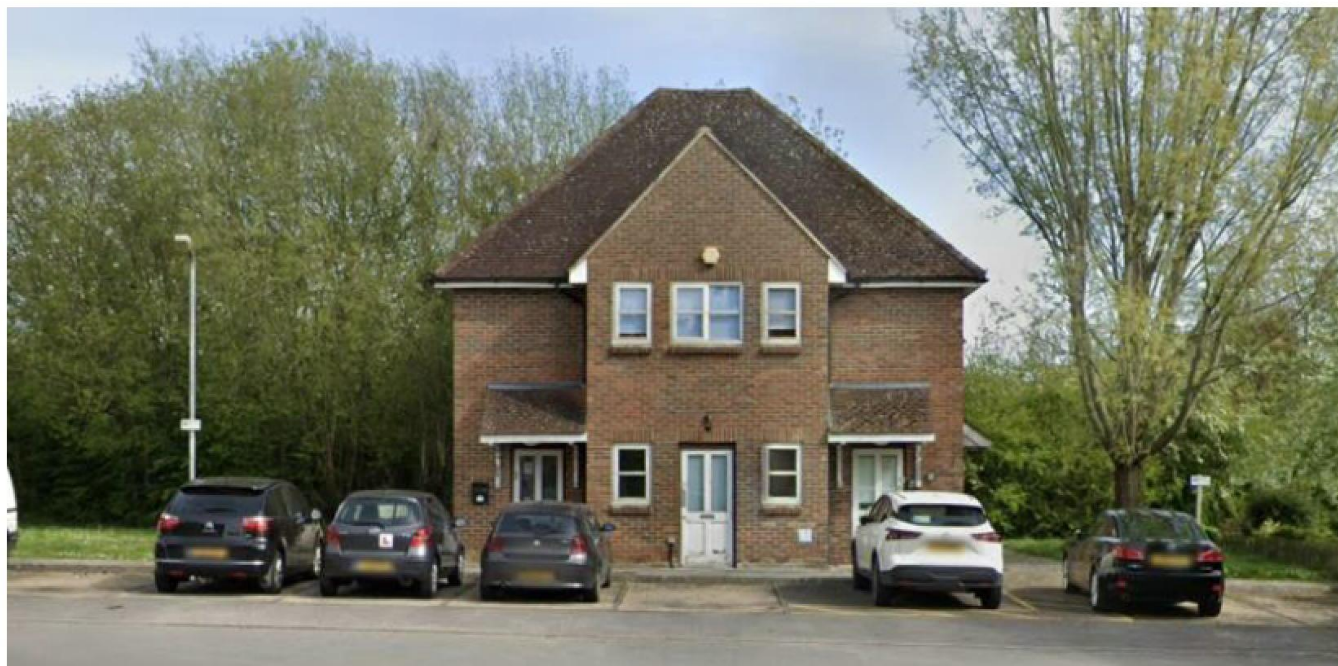
Figure 2- Front Elevation of the Site (Google Maps)
