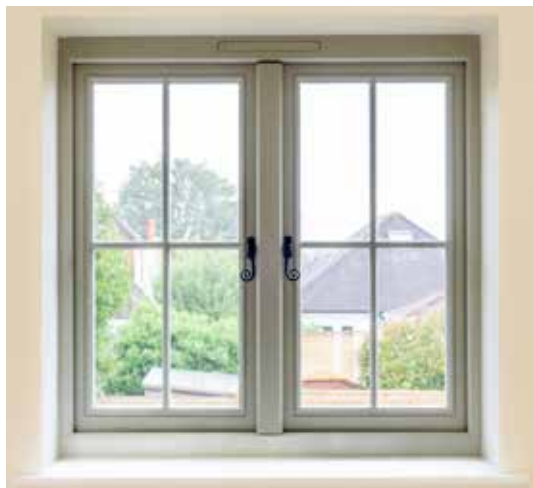
TRICKLE VENT DETAIL
