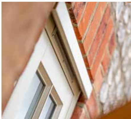
TRICKLE VENT DETAIL
