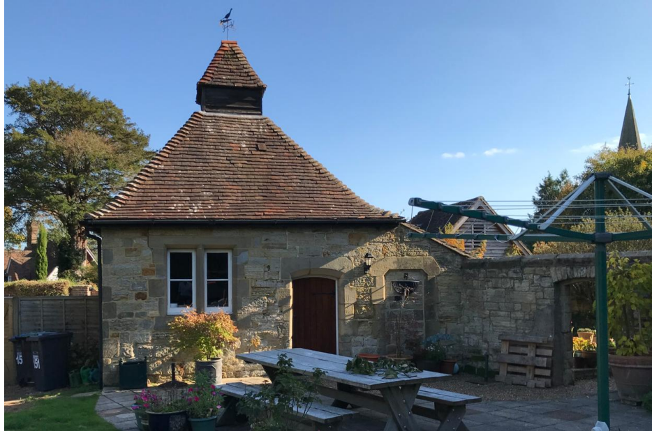
Figure 26: The Bothy (former Bell Tower) viewed from the west
