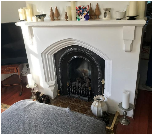
Figure 22: Gothic style painted stone fire surround to left hand ground floor room (Snug) with modern gas fire grate (left) with original stone fire surround and grate to first floor bedroom.
