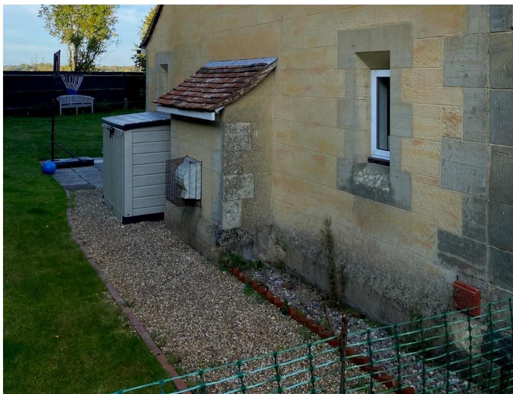
Figure 28: Detail of contrived 'tooled stone' ashlar effect finishes to 1984 extension
