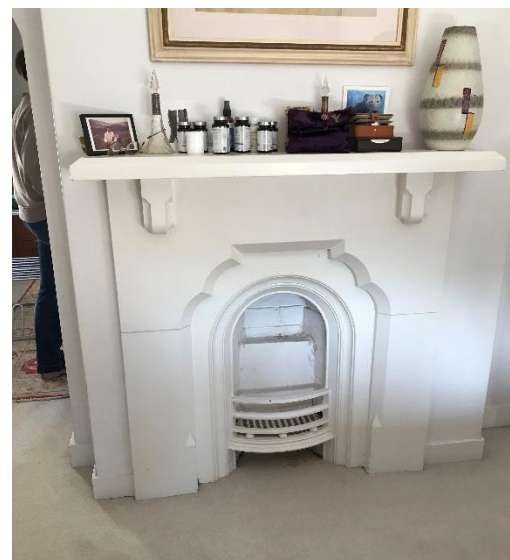
Figure 22: Gothic style painted stone fire surround to left hand ground floor room (Snug) with modern gas fire grate (left) with original stone fire surround and grate to first floor bedroom.
