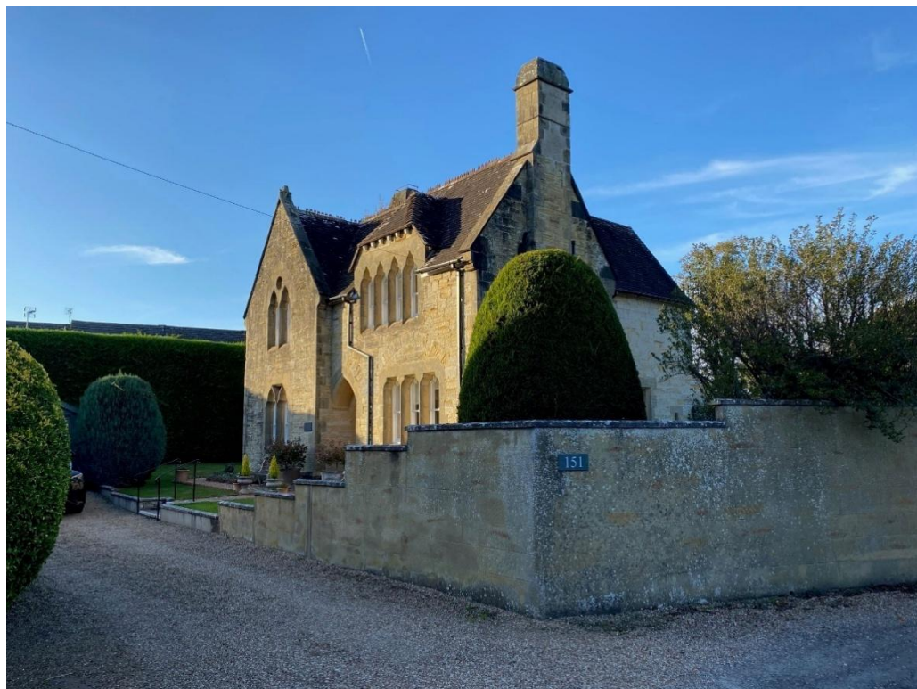
Figure 5: St John's Lodge, viewed from the access drive
