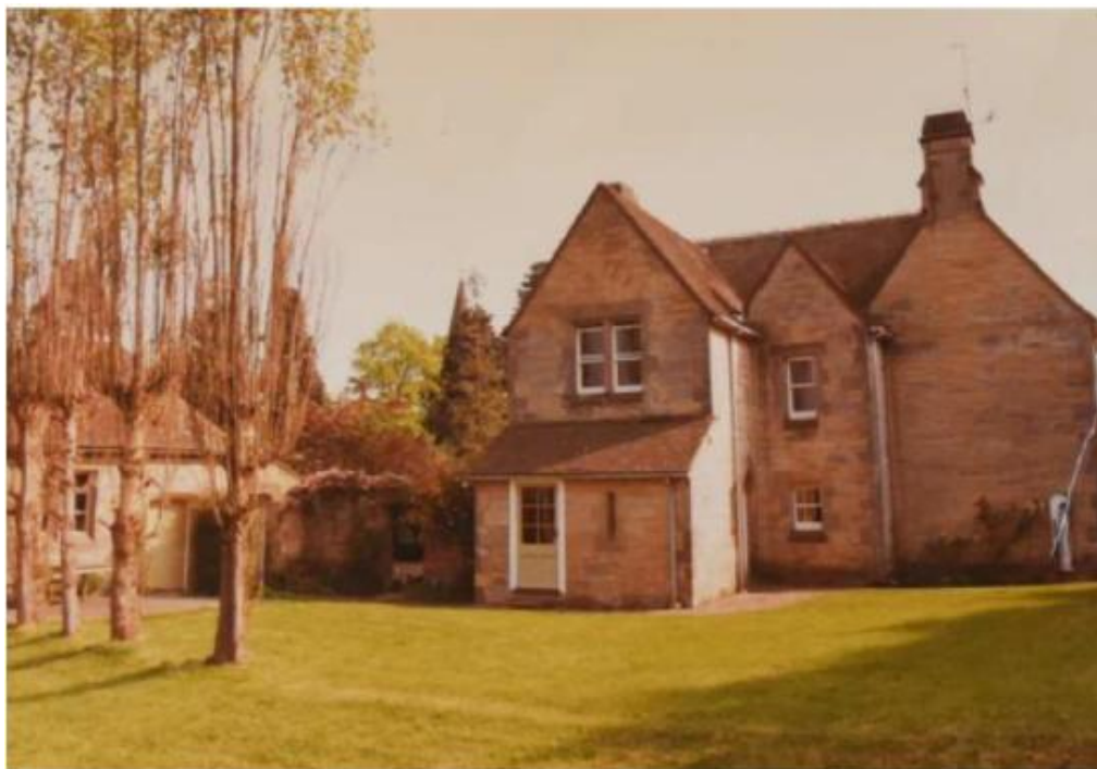
Figure 16: St John's Lodge viewed from the north prior to the construction of the 1984 extension. Source: ASE Heritage Statement
