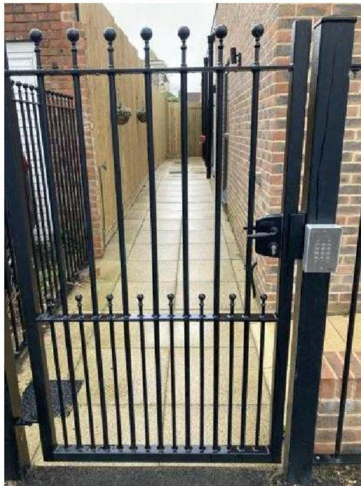
Current back gate; keypad not currently in use
