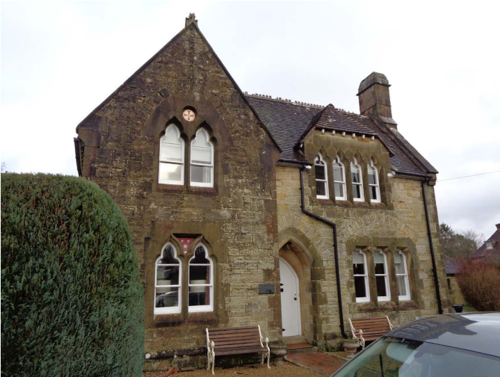
Front (South Western ) View of House
