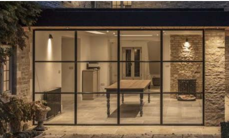
Black metal crittall style glazing doors and windows.
