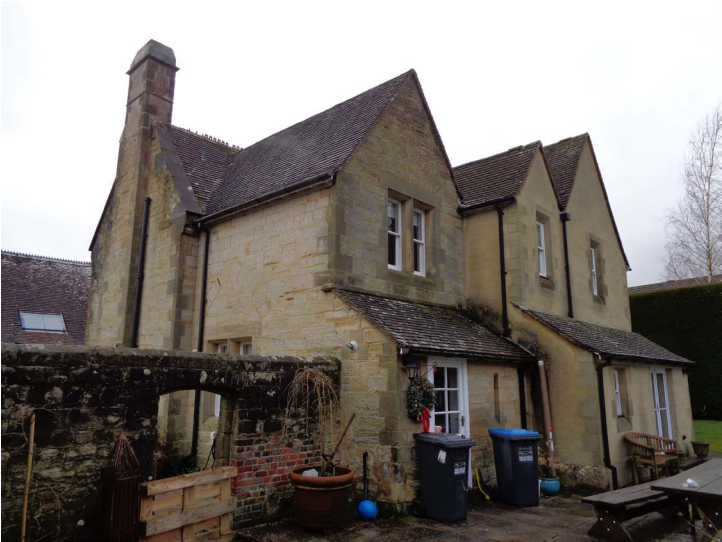
Rear (North Eastern) View of House
