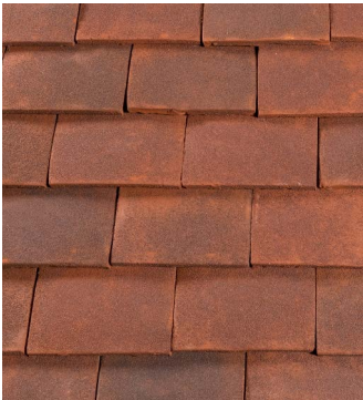
Handmade clay tile roof.
