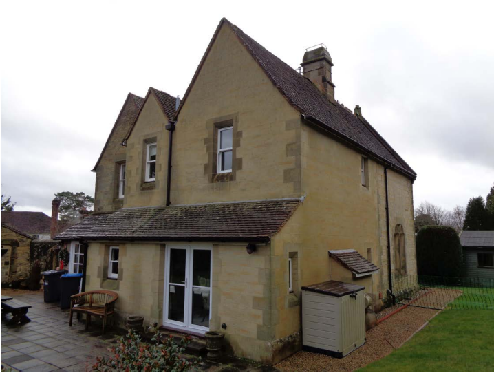
Side (Eastern) View of House
