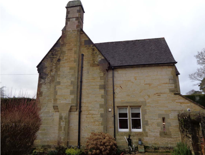
Side (Eastern) View of House
