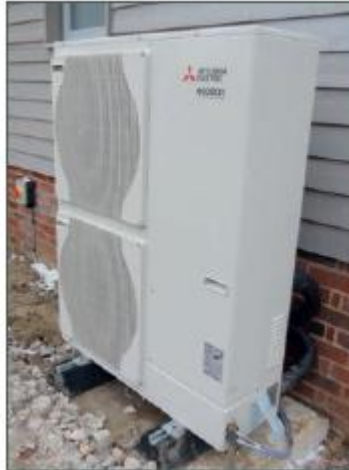
Figure 2 - Typical Air Source Heat Pump
