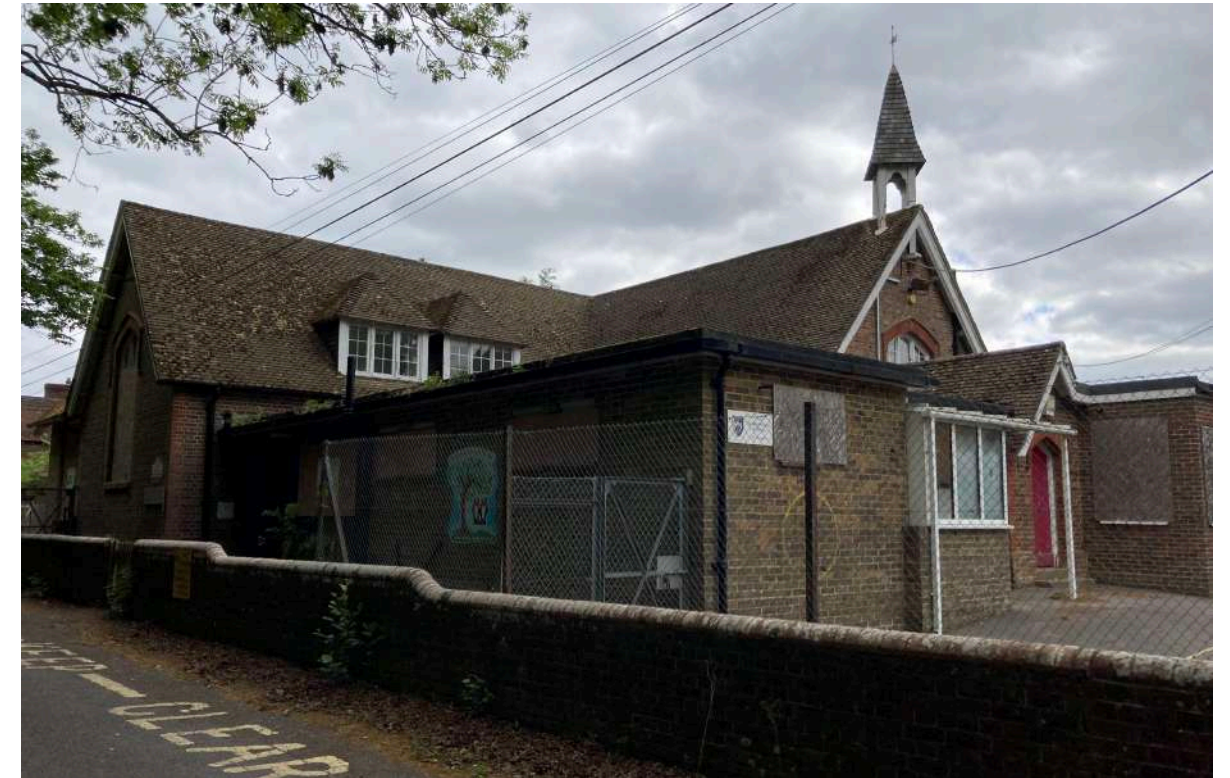
Warninglid Primary School in 2025
