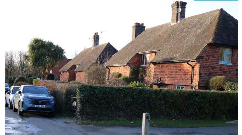
Context Photograph C. Dwellings offset south of the Site along Hoadlands, with ivy cloaked box and beech hedge.
