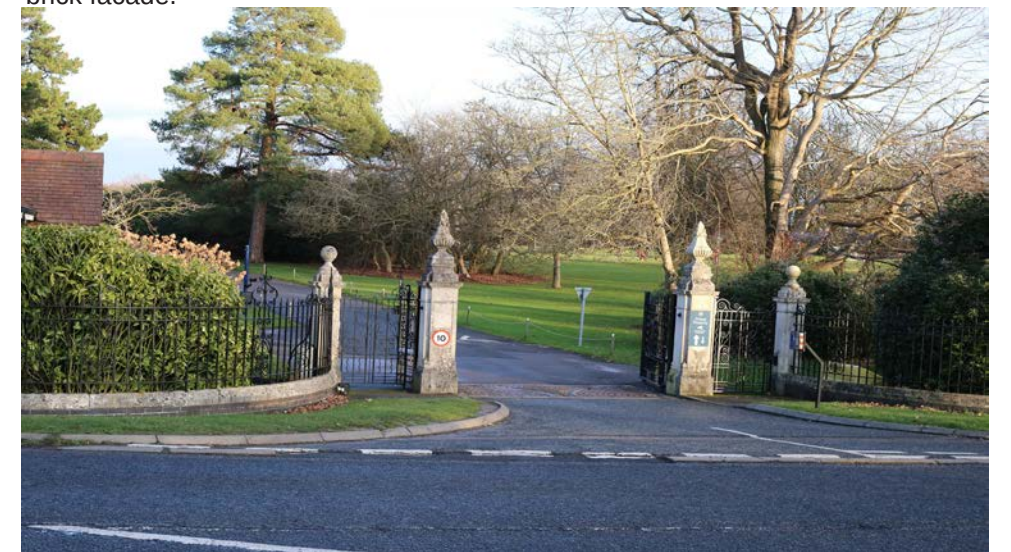
Context Photograph I. Ornate stone pillars to either side of the private gateway entrance to Handcross Park School.
