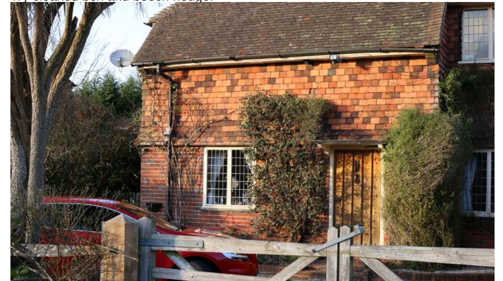
Context Photograph F. Hoadlands property - Showing mottled tile hung and brick facade.
