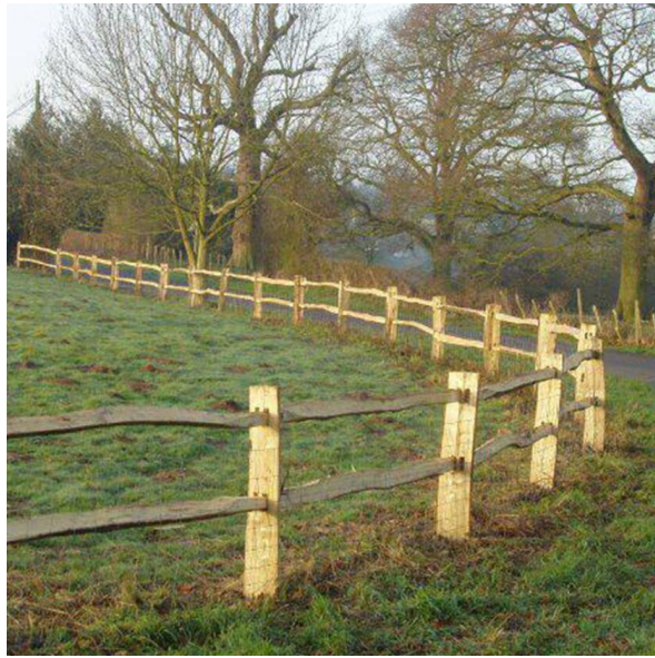
Post and rail fencing
