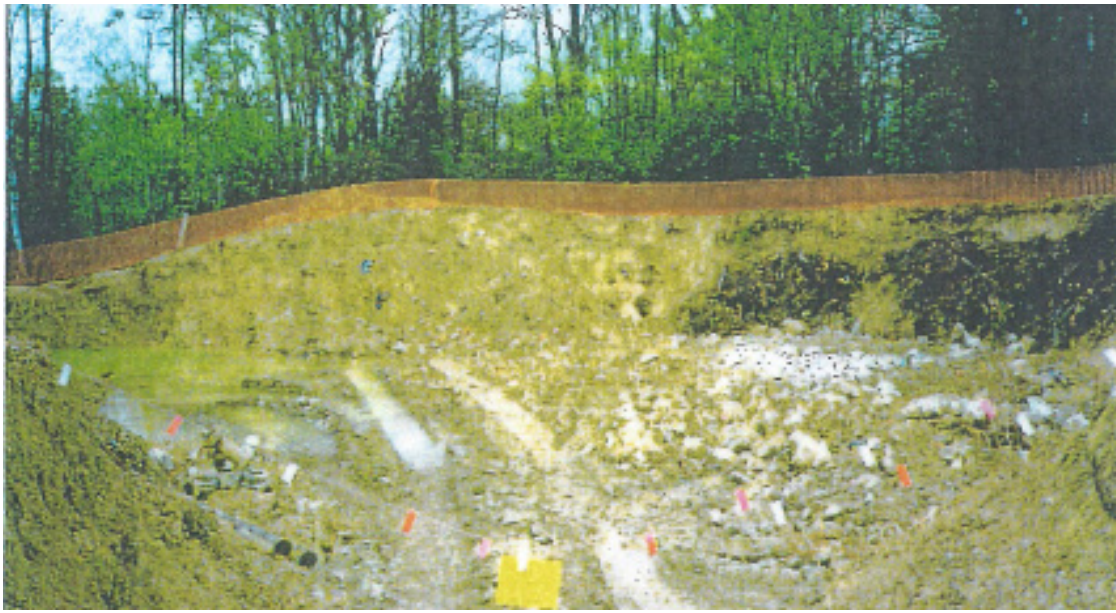
Small Tank after removal of concrete walls - South
