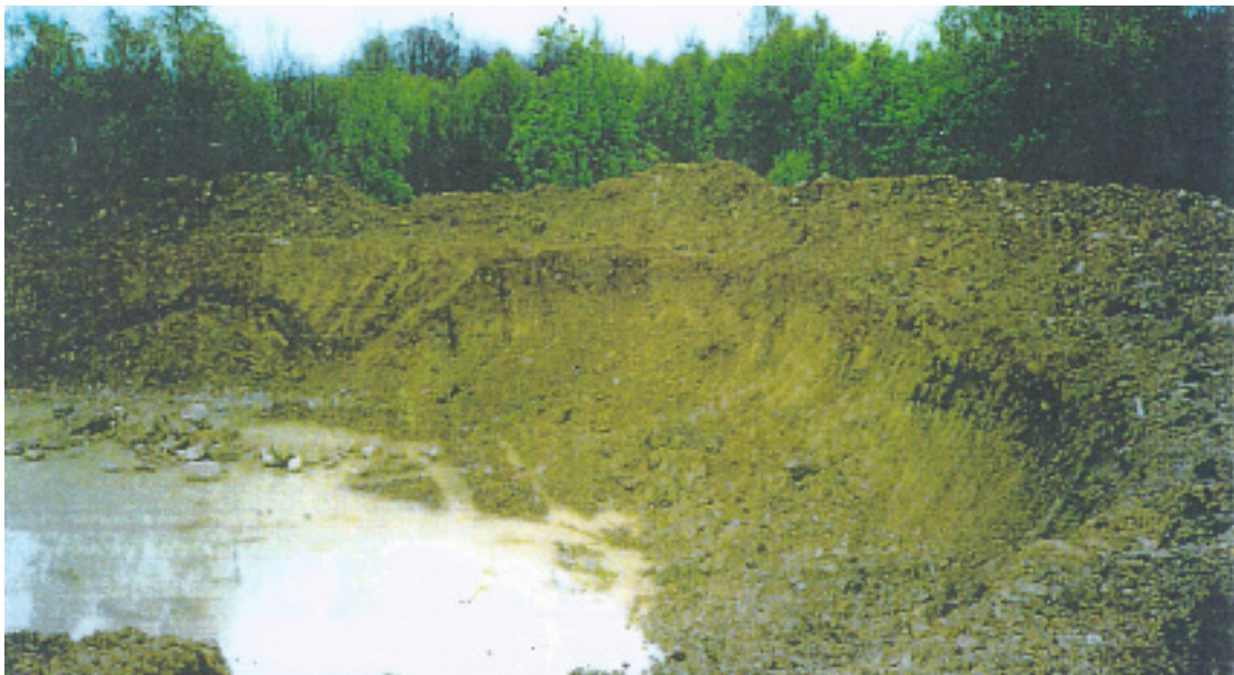
Large tank after removal of concrete walls - concrete base remains
