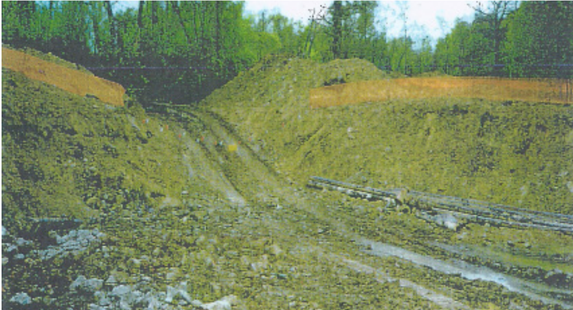
Small Tank after removal of concrete walls - North
