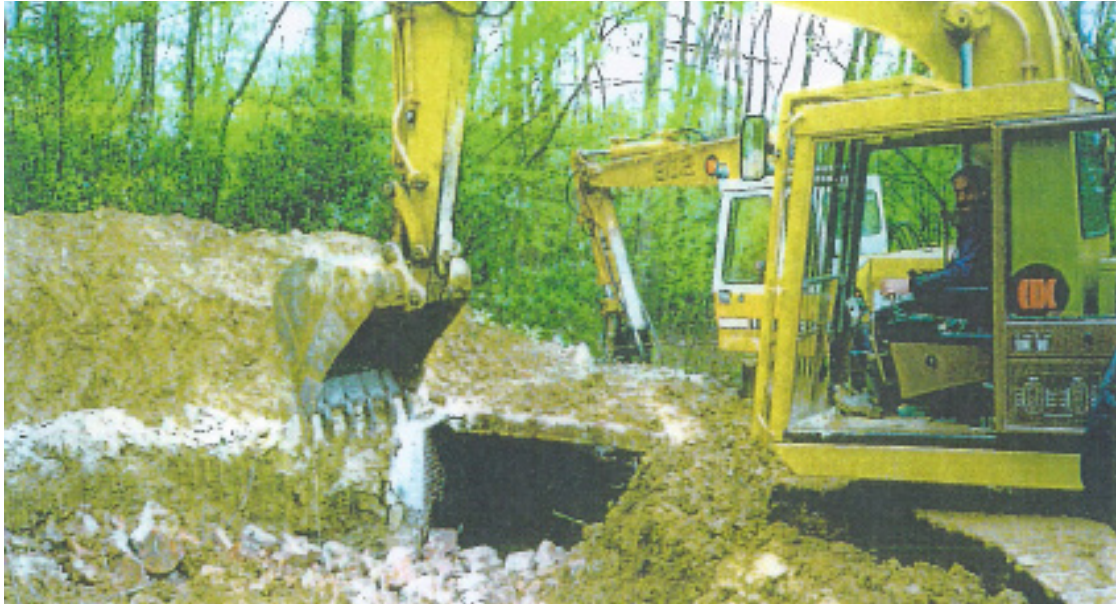
Removal of Entrance to Small tanks
