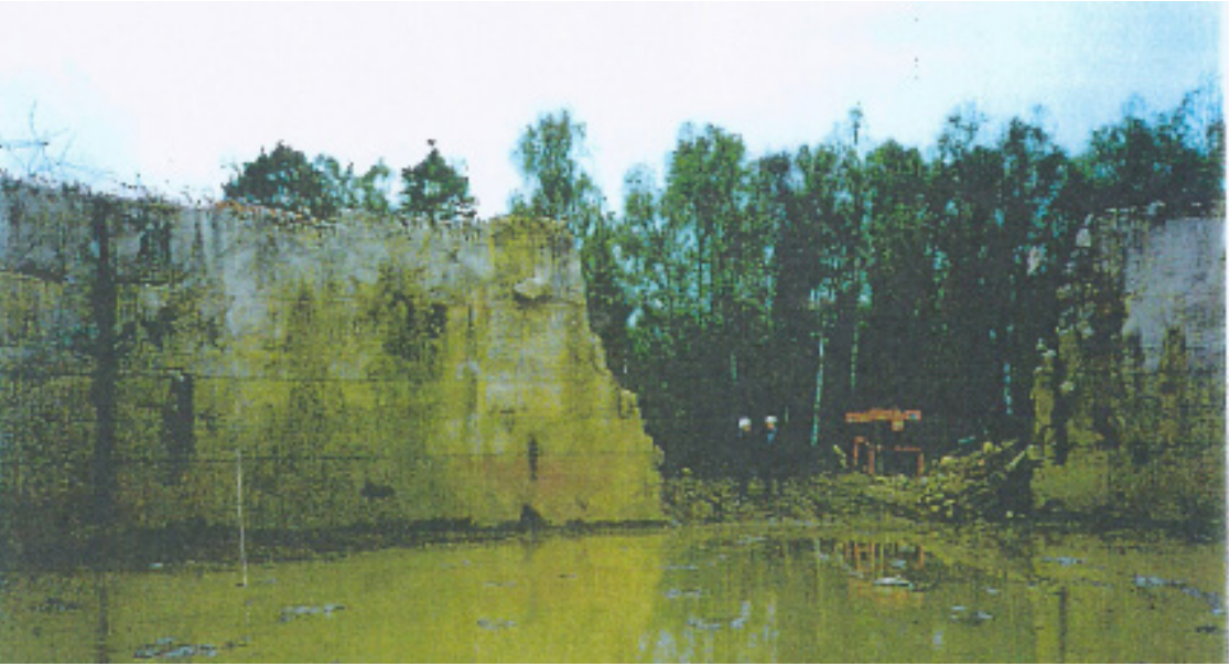
View inside large tank showing concrete walls with steel removed
