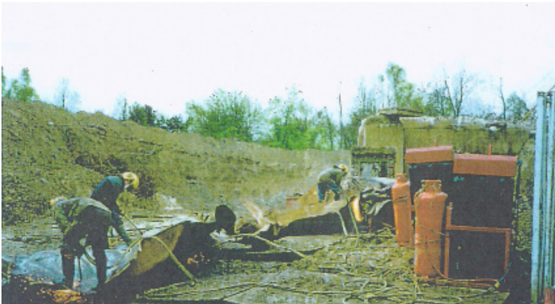
Cutting the steel of the Large Tank
