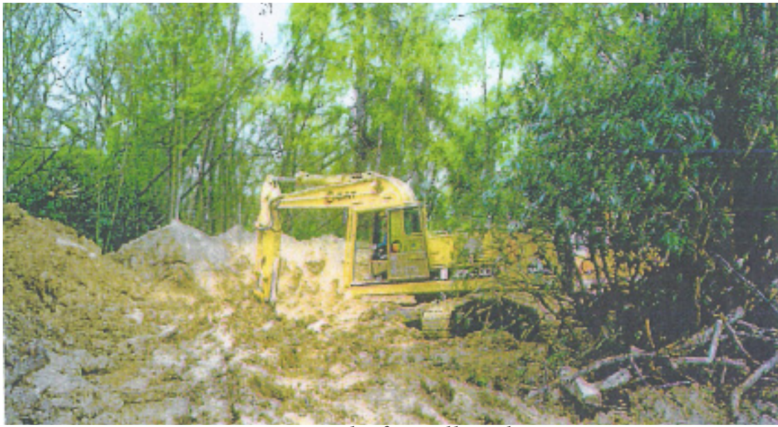
Removal of Small tanks
