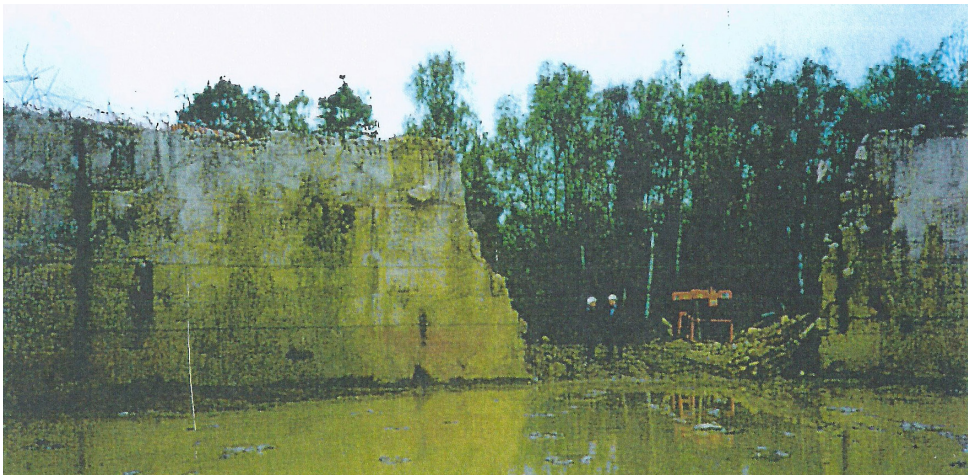
View inside storage tank showing concrete walls with steel removed
