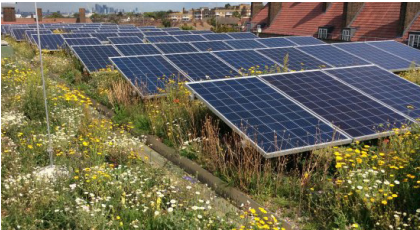
Hybrid Blue, Green & Solar Rooftop (Biosolar)
