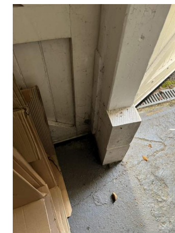
8 Repair splice to base of timber post
