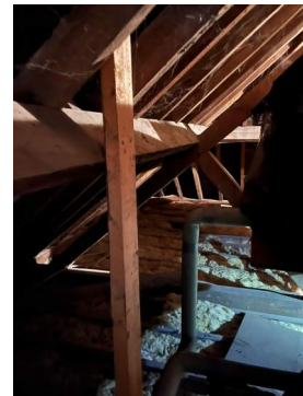
3 Typical addition roof framing
