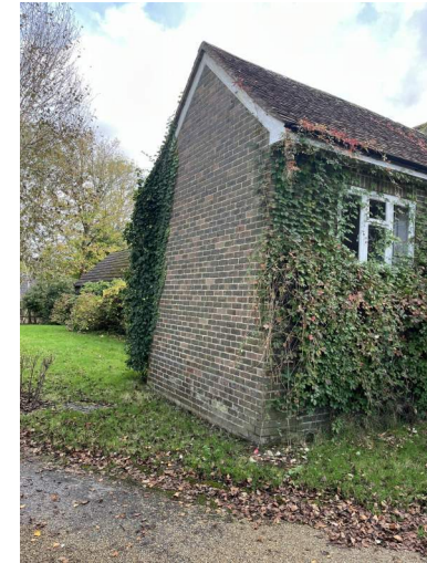
3 Gabled extension; appears to be a later addition in cavity masonry
