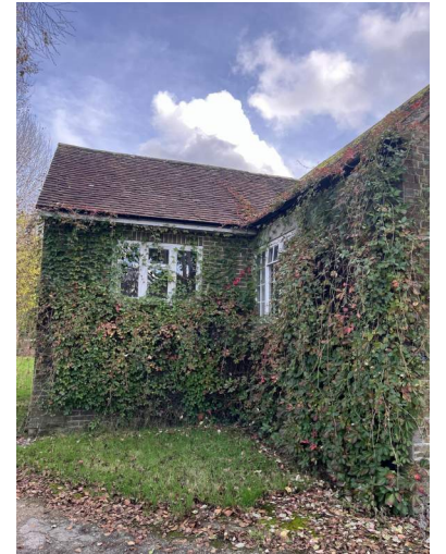
4 Extension - roof hipped onto original
