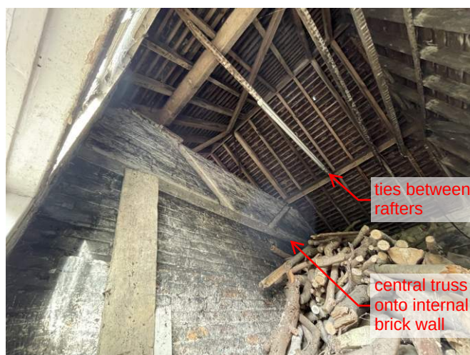
8 Southern side internal wall
