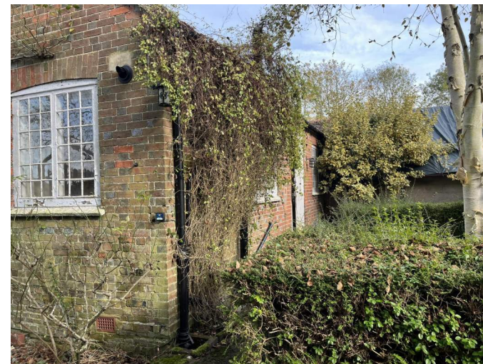
7 Southern elevation facing garage
