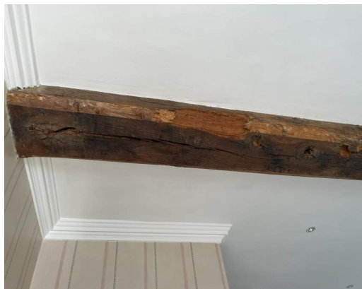
7 Downstand timber beam
