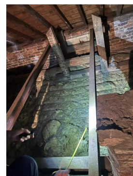
14 Suspected support structure to early clock
