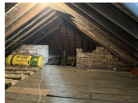
15 Original external wall parapet with later roof addition beyond
