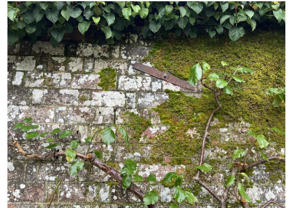
4 2no. ties / pattress plates in wall
