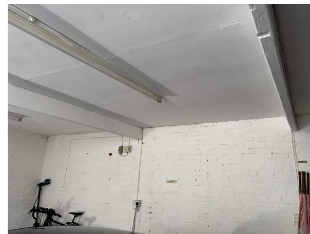
7 Downstand beams bear into rear elevation masonry
