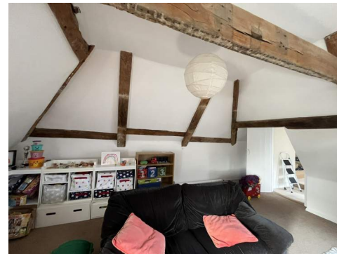
4 Original early main house roof framing
