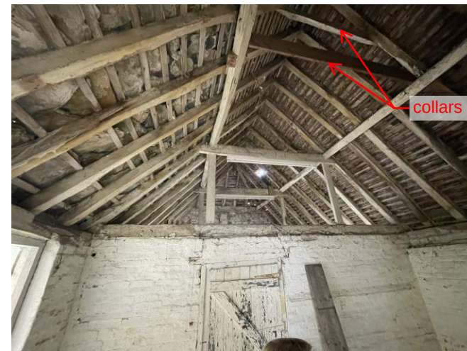
5 Timber framing & internal wall
