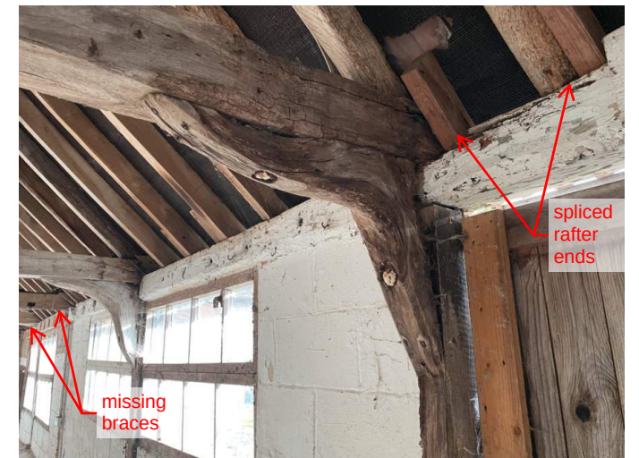
9 Typical timber framing on southern wall
