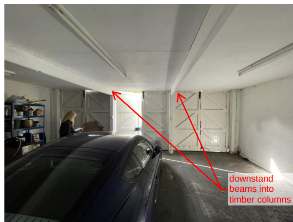
6 2no. downstand beams into timber columns
