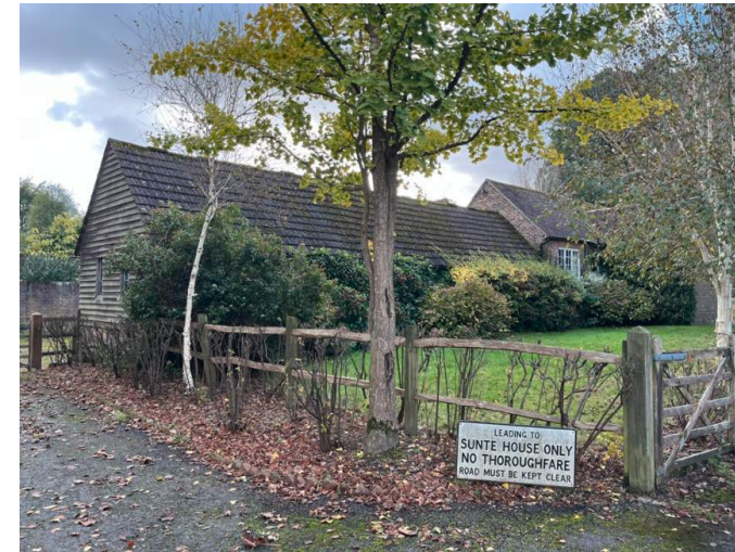
3 Northern elevation with extensive vegetation & Cottage gable wall
