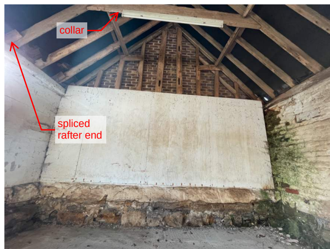
6 Original timber framed stable external wall, cottage wall built against stables
