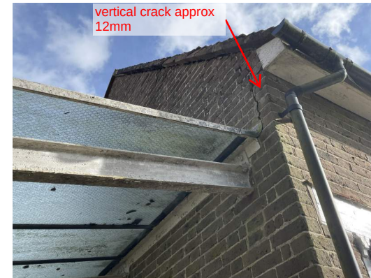
3 External cracking
