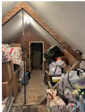
1 Late C19th addition roof truss
