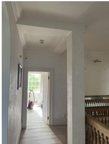
1 Boxed out downstand beam & column
