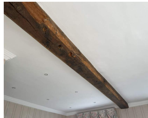
8 Downstand timber beam
