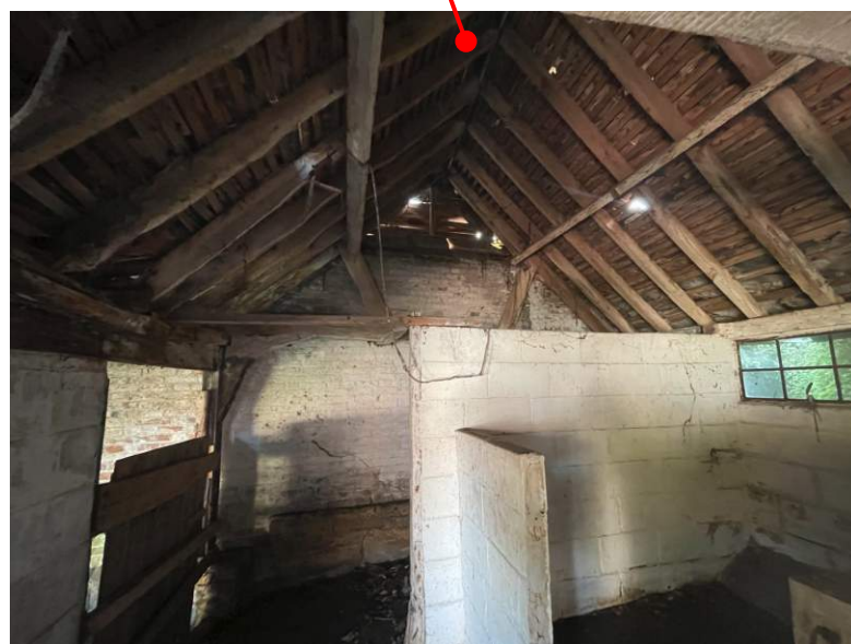
3 Byre end gable wall
