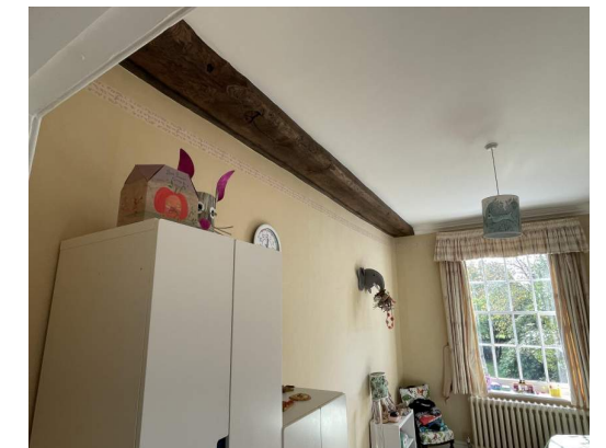
11 Non-load bearing partition built to underside of downstand timber beam
