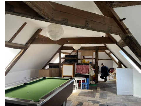
5 Staggered butt purlin roof with oak pegged tenons
