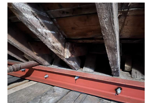
18 PFC either side of timber
