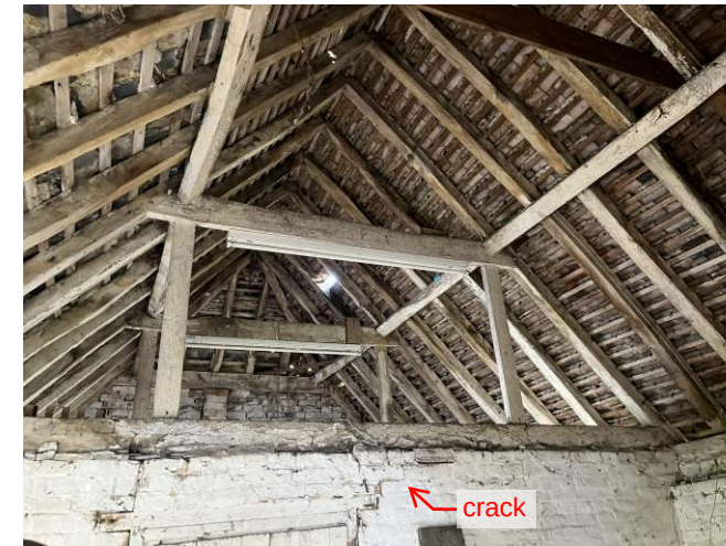
3 Internal dividing wall with timber framing over
