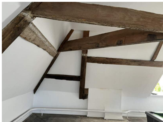
8 Hip truss framing
