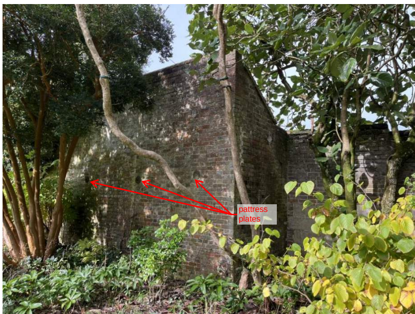
3.1 Pattress plates visible on external southern wall of Garden Store
