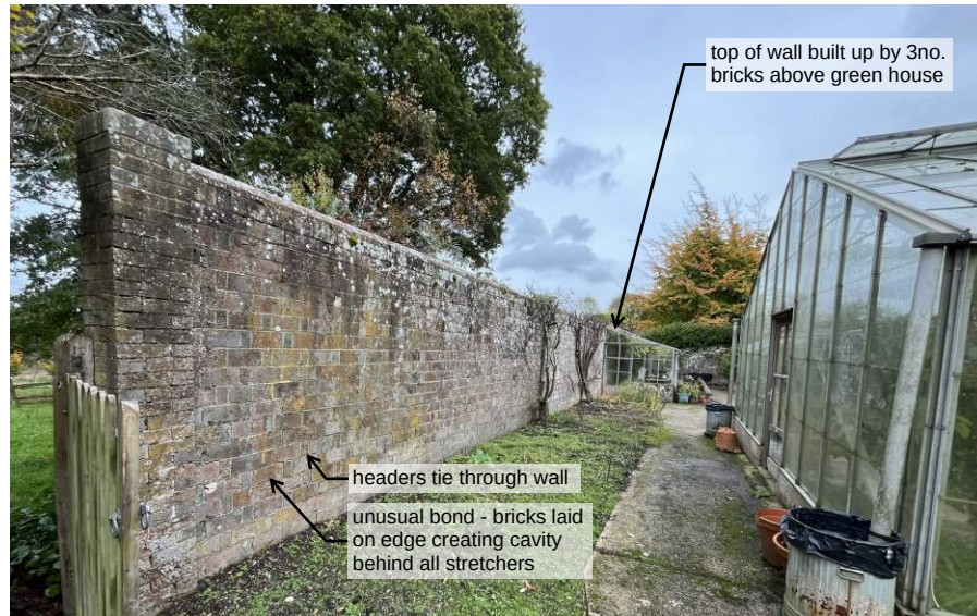
1 Wall behind green houses, to form rear wall of swimming pool building
