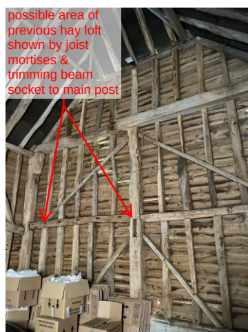
8 South gable wall
