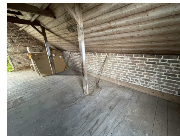
12 Remedial struts & timber structure
