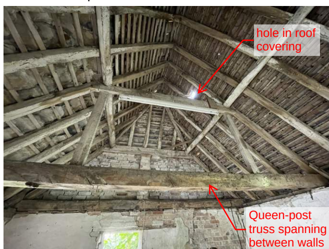
8 Internal timber queen post truss
