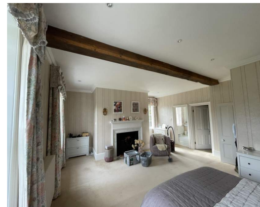
9 Downstand timber beam
