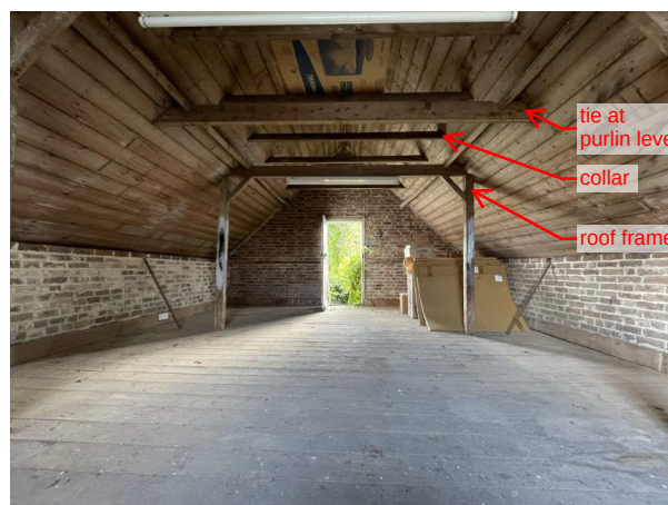
10 1st floor & roof framing
