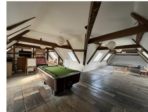
6 Principle rafters, purlins & ties partially visible below plaster
