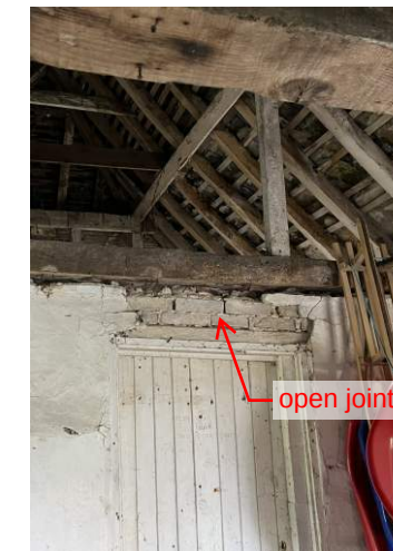
7 Lintel in internal wall
