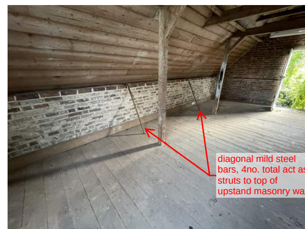
11 Historic ties from roof to floor
