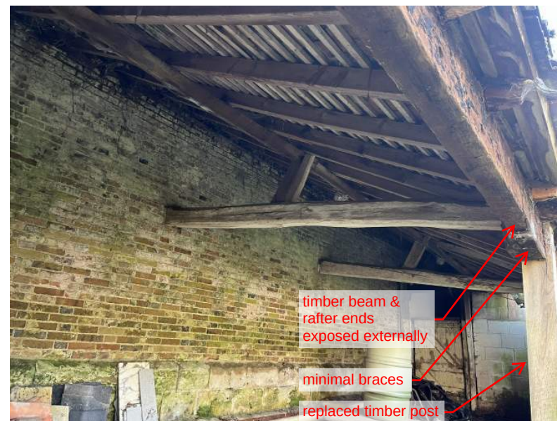
6 Typical roof construction & rear wall
