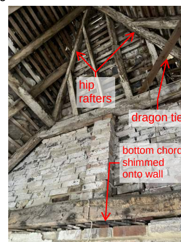
9 Northern gable end wall
