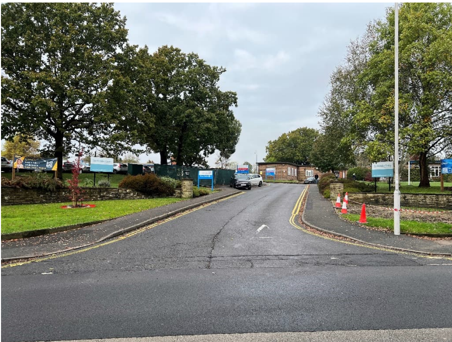
Figure 3-1: QVH Main Gate
