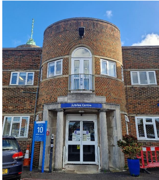
Figure 4.6: Main entrance to the Jubilee Building on the north-western façade
