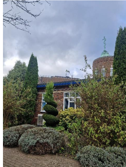
Figure 4.8: Planting adjacent to the south-eastern façade of the Jubilee Building
