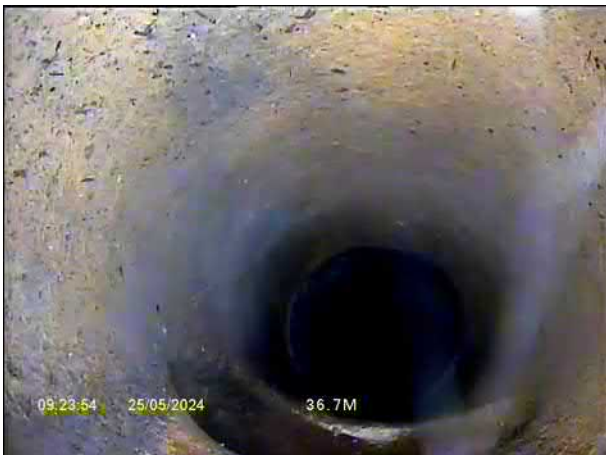
00:04:38, 36.70 m Junction at 6 o'clock, diameter: 150mm, Drop shaft
