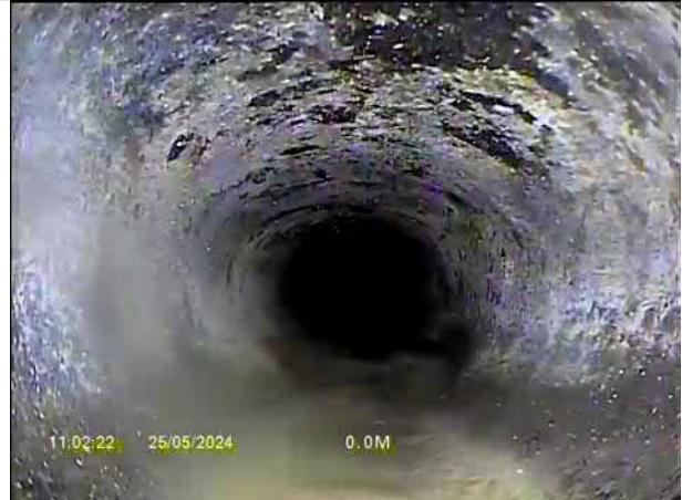
00:00:13, 0.00 m Water level, 0% of the height
