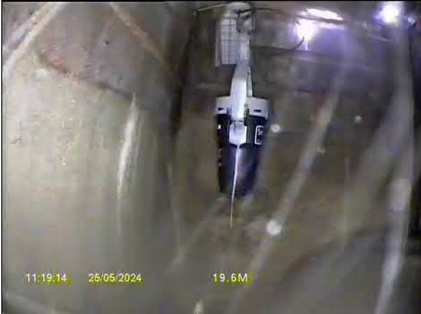
00:01:39, 19.50 m Finish manhole, MH05/5902, the pipe is flowing fine
