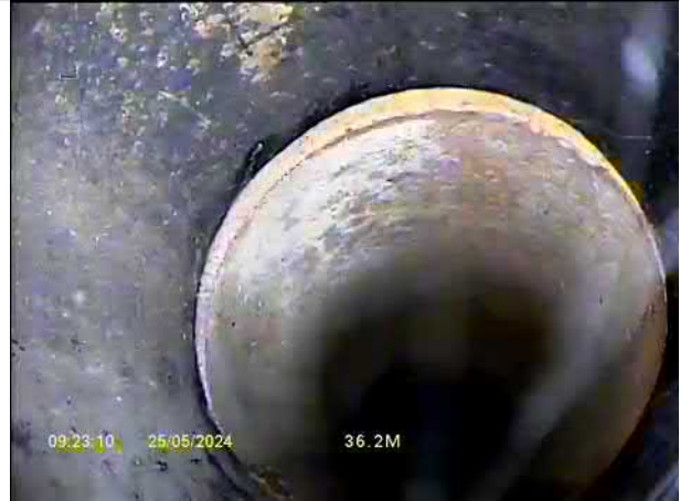
00:03:55, 36.20 m Pipe material changes, to vitrified clay
