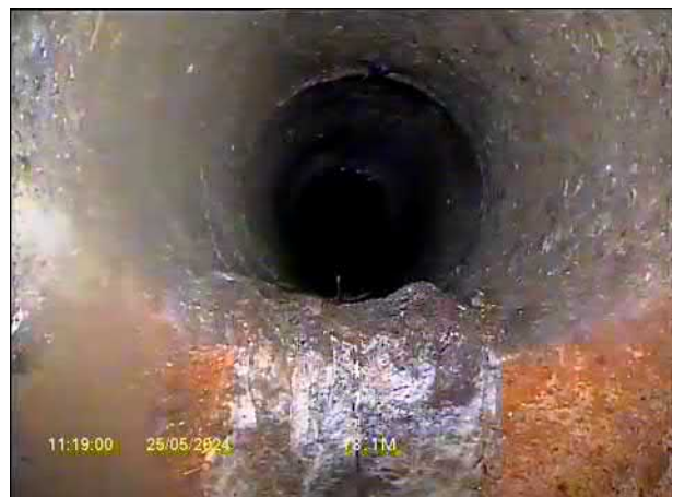
00:01:24, 18.10 m Junction at 6 o'clock, diameter: 150mm, Drop shaft
