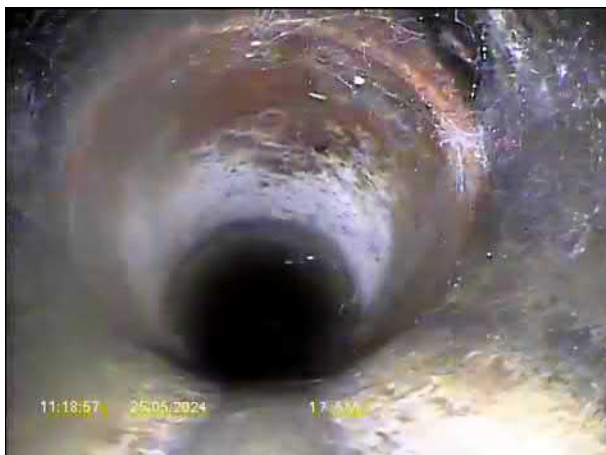
00:01:21, 17.60 m Pipe material changes, to vitrified clay
