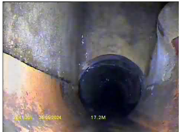
00:02:09, 17.20 m Finish manhole, MH03/5803, the pipe is flowing fine
