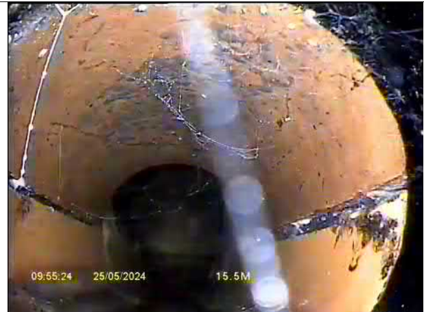
00:03:29, 15.40 m Pipe material changes, to vitrified clay
