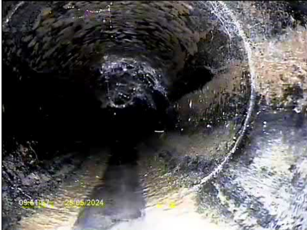
00:00:00, 0.00 m Start manhole, MH5801
