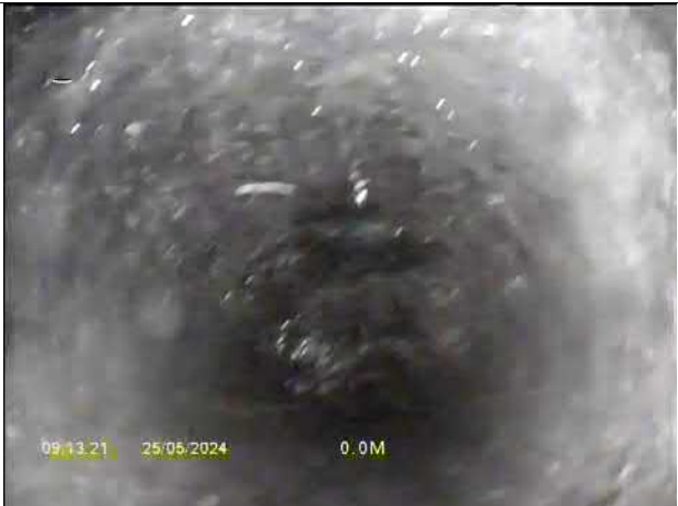
00:00:23, 0.00 m Water level, 0% of the height
