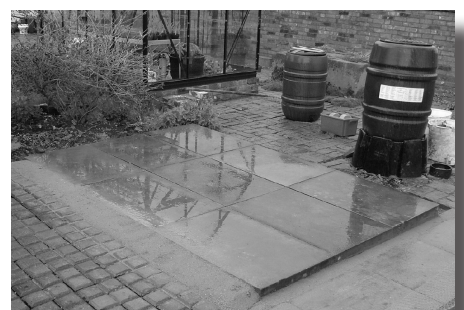
A 6x8 slab base: ideal for a 5x6 greenhouse. Remember that your greenhouse is a few inches bigger than the nominal size.
