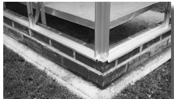
A brick base must be made to the exact millimeter stipulated by the manufacturer's base sizes because the cill overlaps the brick.
