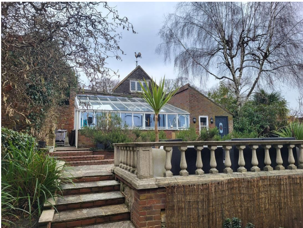
Plate 10: Looking north across No.19's rear garden towards boundary with Estcots Barn. The boundary wall behind the conservatory is historic; beyond this the gable end of an outbuilding associated with the barn can be seen
