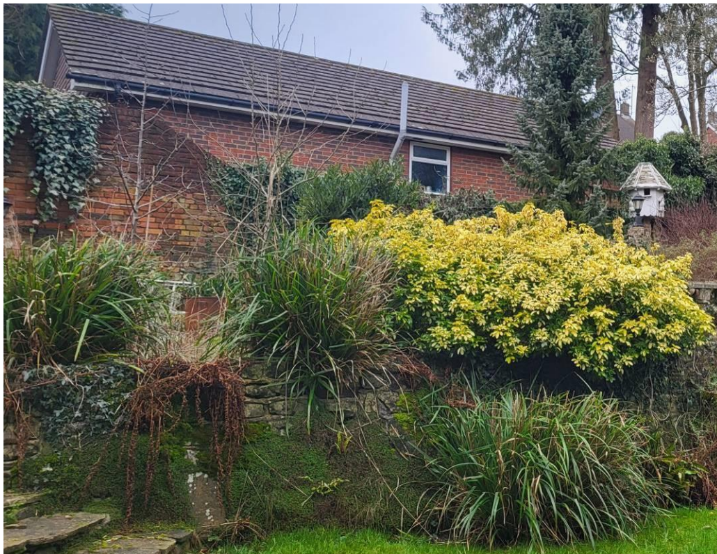
Plate 8: Section of western boundary wall of application site (to left), with No.17 Estcots Drive beyond
