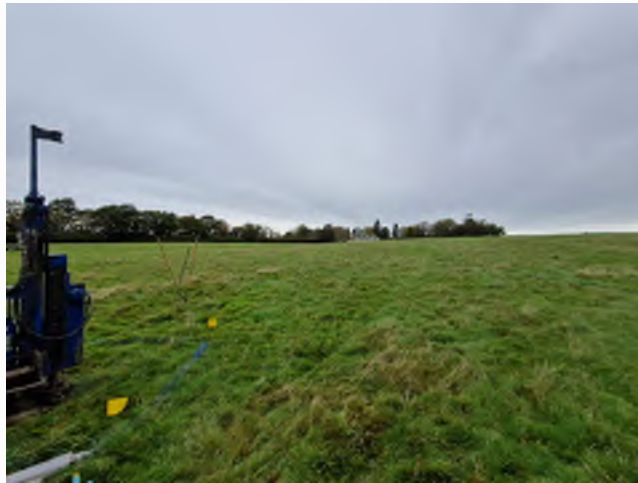
View from West facing East
