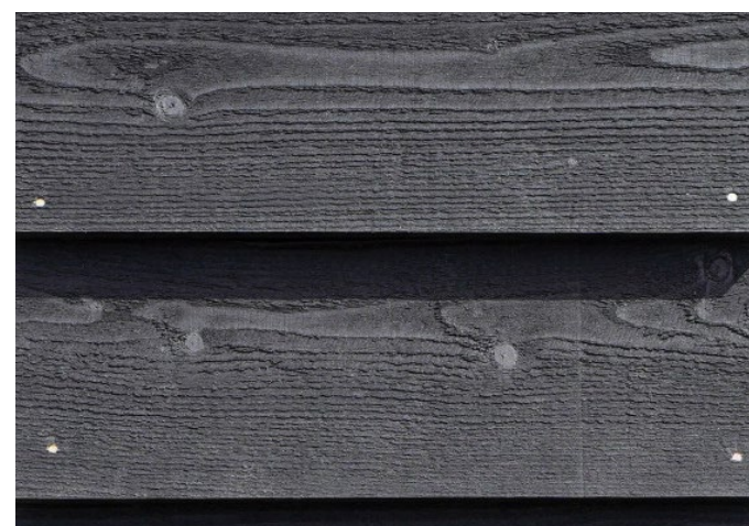
Walls - Black Feather Edge Cladding (Close Up)
