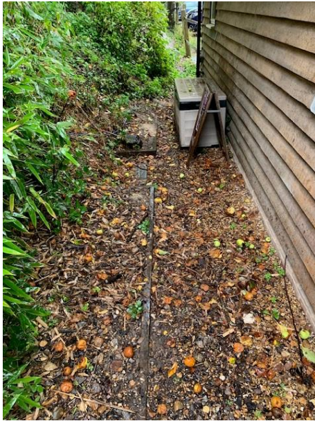
Photo 2 – Location of utilities run behind existing Visitor Reception building
