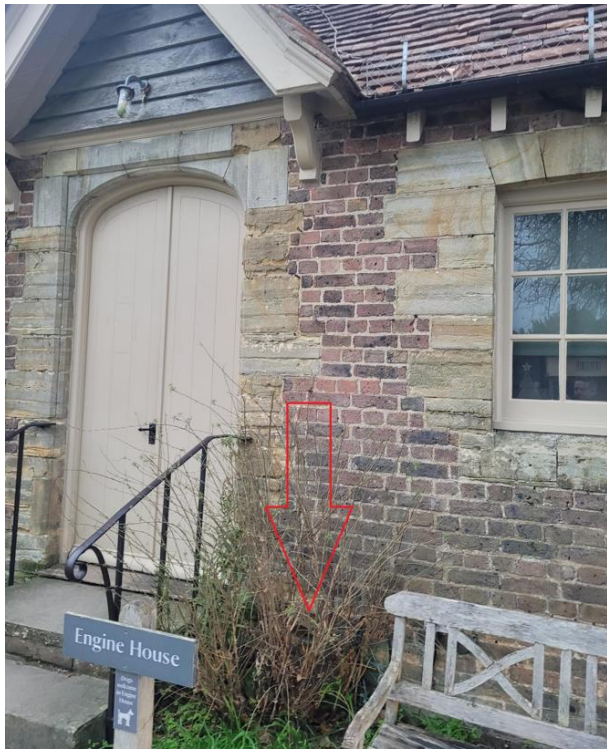
Photo 9b – Approximate location of insertion point for water pipe (red arrow).
