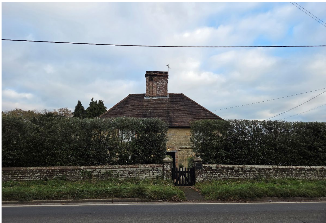
Plate 7. Grade II Listed Cleavewater
