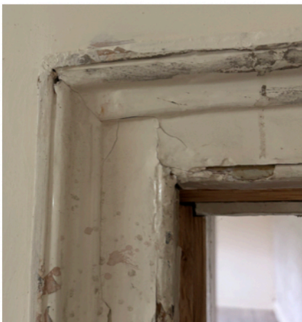
Existing architrave - all new to match
