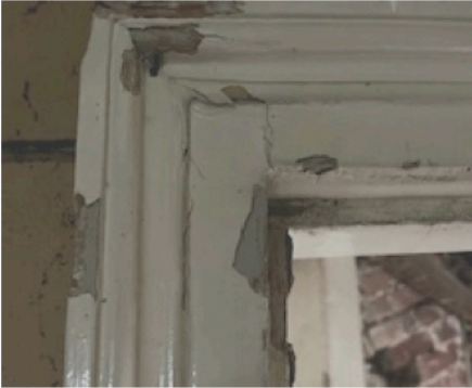
Existing architrave - all new to match
