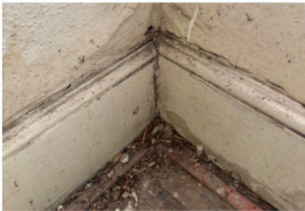
Torus skirting board - all new to match existing
