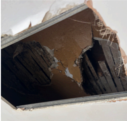
G.05 - Suspended ceiling.
