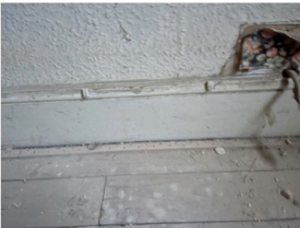
Torus skirting board - all new to match existing
