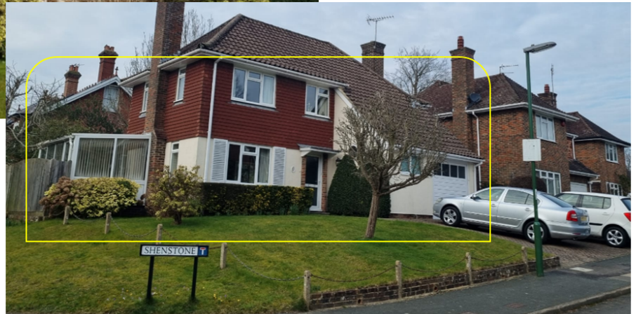
Diagonally opposite The Slatch. Basic uPVC Conservatory and windows... on Hickmans Lane. Visible from 'The Barn'
