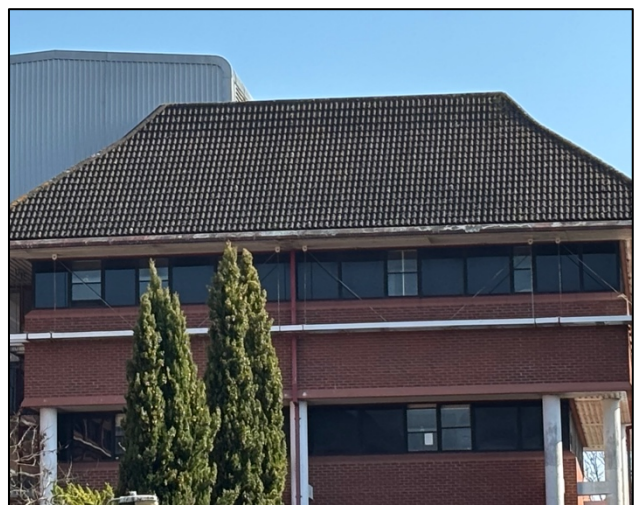
Photograph 3a and 3b. Example of the tiled roof hips on the outer edges of the building.
