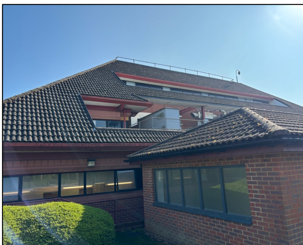
Photograph 3a and 3b. Example of the tiled roof hips on the outer edges of the building.
