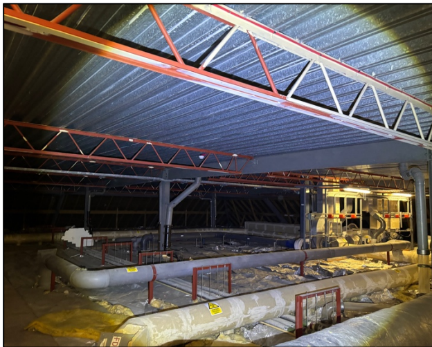
Photograph 2a and 2b. Example of the roof voids scattered across the top floor of the hospital, including services infrastructure (left) and the underside of the bitumen-lined tiles (right).
